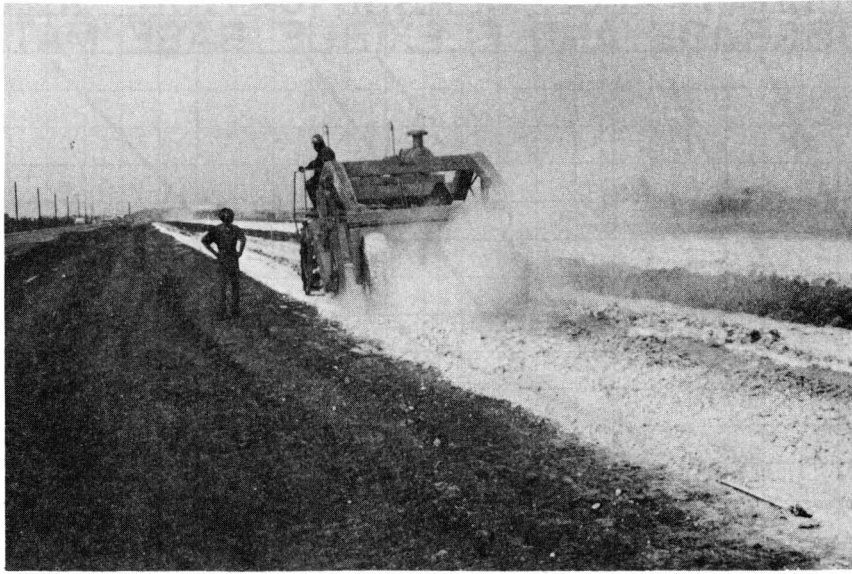
Photograph 7. Beginning of Mixing of Pelletized Lime.
