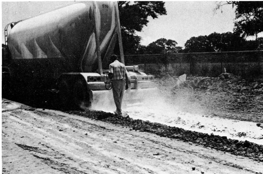
Photograph 2. Showing Close Up View of Pelletized Lime Distribution.
