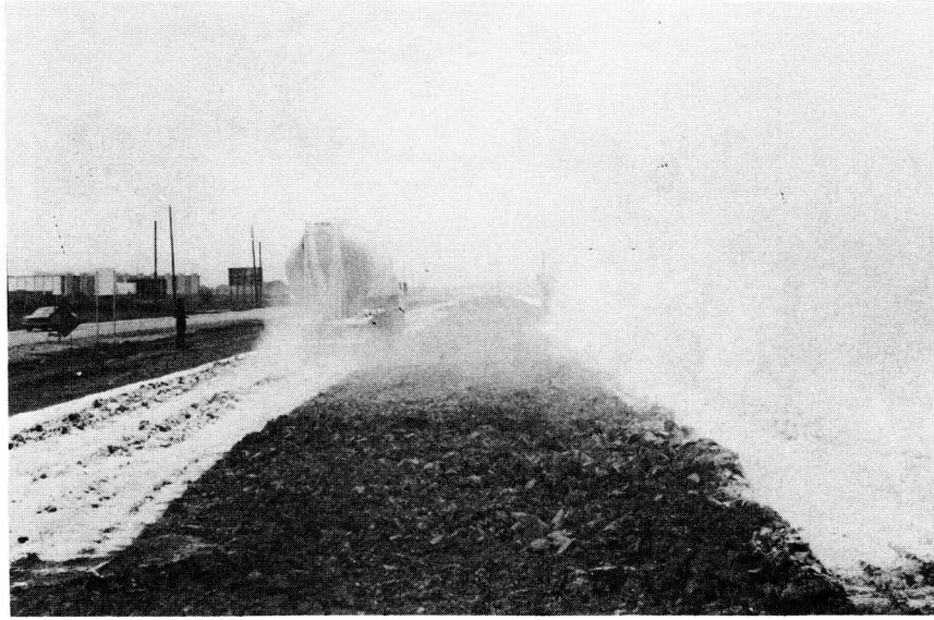
Photograph 5. Showing Dusting of Hydrated Lime on U. S. 59 Near Houston.
