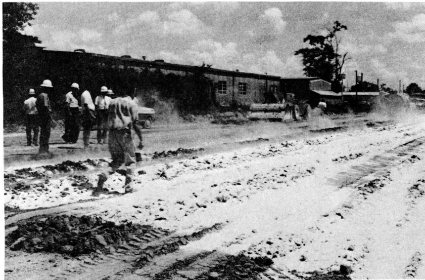
Photograph 4. Showing Steaming of Quicklime in Pelletized Lime After Sprinkling.
