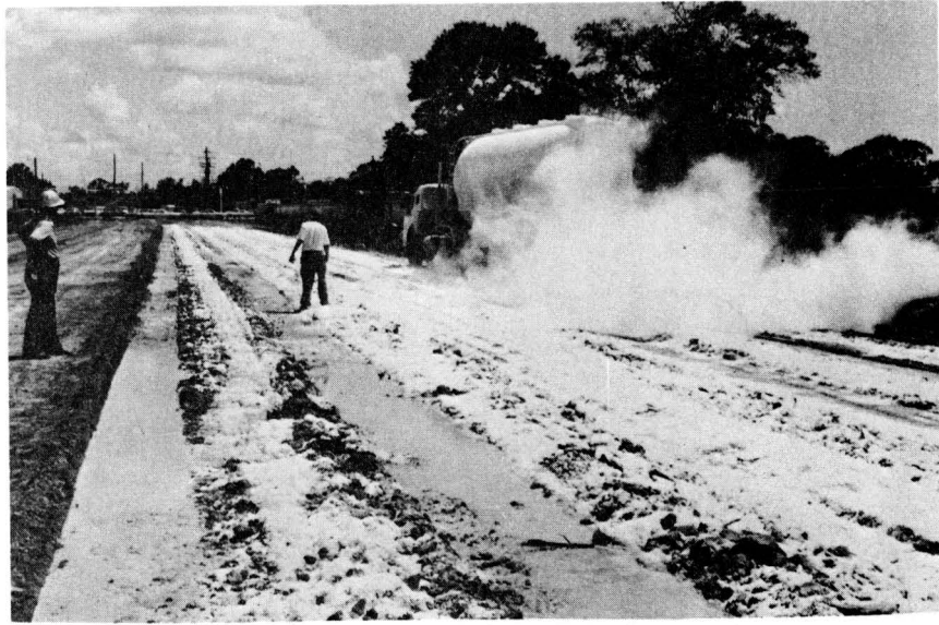
Photograph 3. Showing Pelletized Lime Dusting Upon Nearing Final Emptying of Truck.
