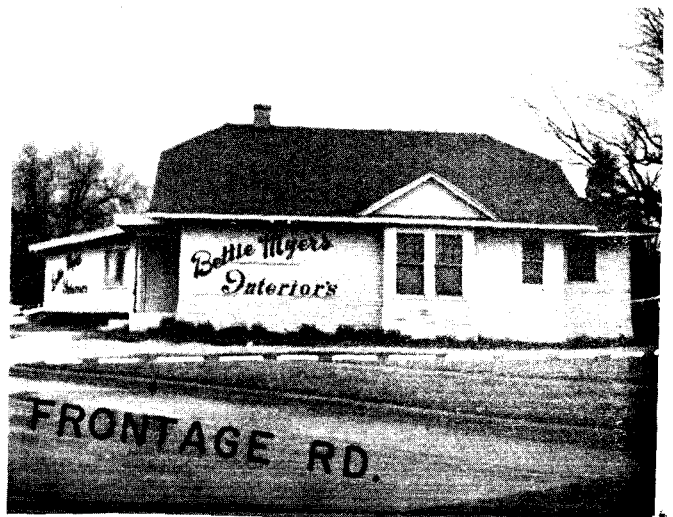
FRONTAGE RD. 2 - AFTER ACQUISITION.
