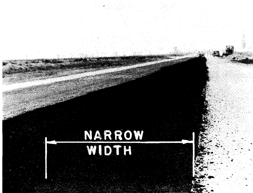
NARROW WIDTH SPREAD BY BLIND-HEEL PASS
