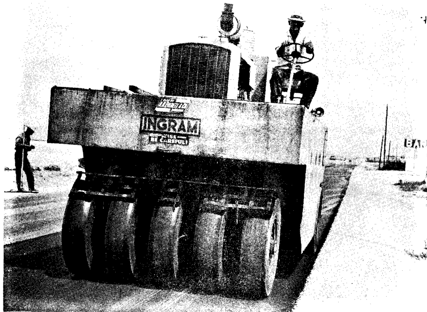
SHOWING PNEUMATIC ROLLER
