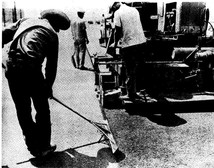
SHOWING OVERLAP OF LONGITUDINAL JOINT BY PAVER SCREED
