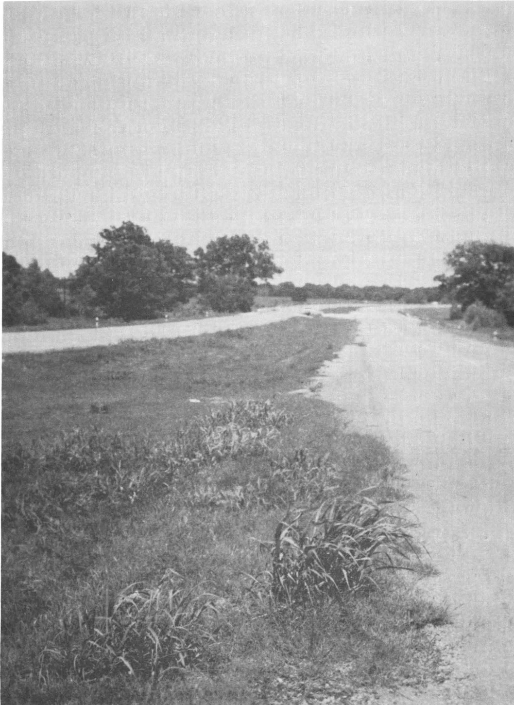
Figure 1. Paved shoulders which carry little or no traffic are often invaded by Johnsongrass, Bermudagrass, and other vegetation.
