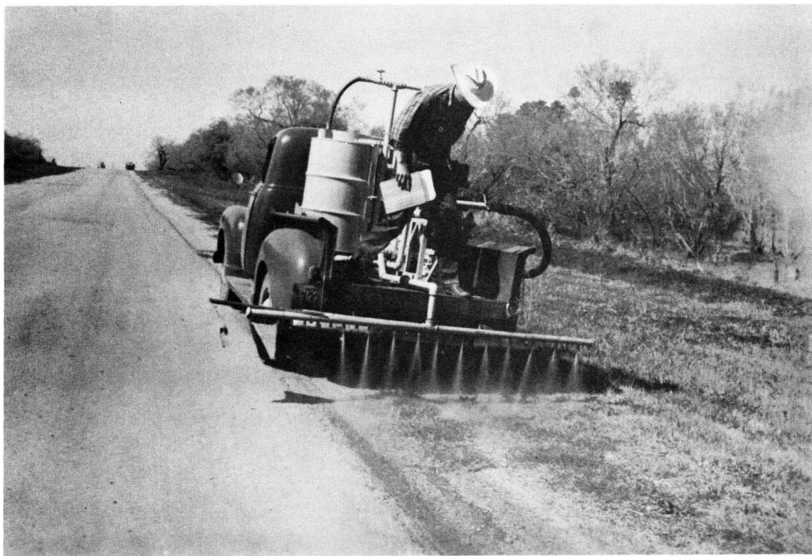
Figure 4. (Above) The spray pattern from the fan type nozzle is easier to use than either the hollow cone (shown above) or the solid cone. In practice the fan nozzle tip can be turned so that the spray from one nozzle does not interfere with spray from the next nozzle on the spraybar. Also, the nozzle tips which produce the fan pattern can be set at whatever angle to the direction of travel is needed to give a uniform coverage across the swath (below).
