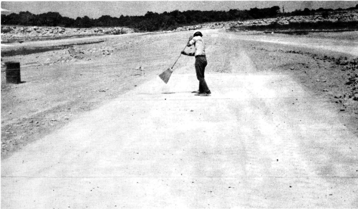
Figure 12: SWEEPING PAVEMENT TO EXPOSE CRACK PATTERN
