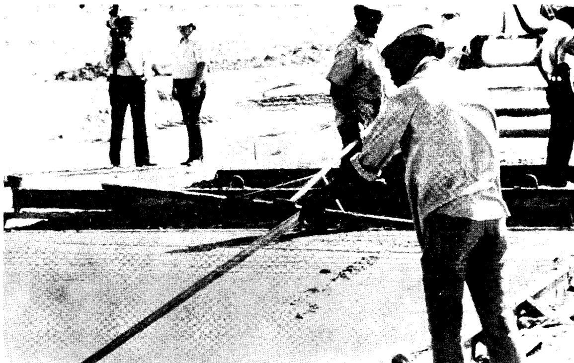
Figure 7: PLACEMENT AND FINISHING WERE RELATIVELY EASIER AT \frac{V_r}{V} = 0.97\%
