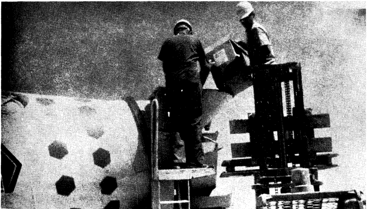
Figure 5: GLASS RIBERS ADDED TO READY-MIX AT THE JOB SITE
