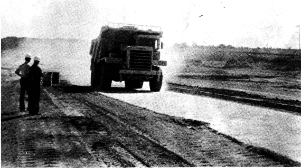
Figure 11: FIRST TEST LOAD APPLIED
