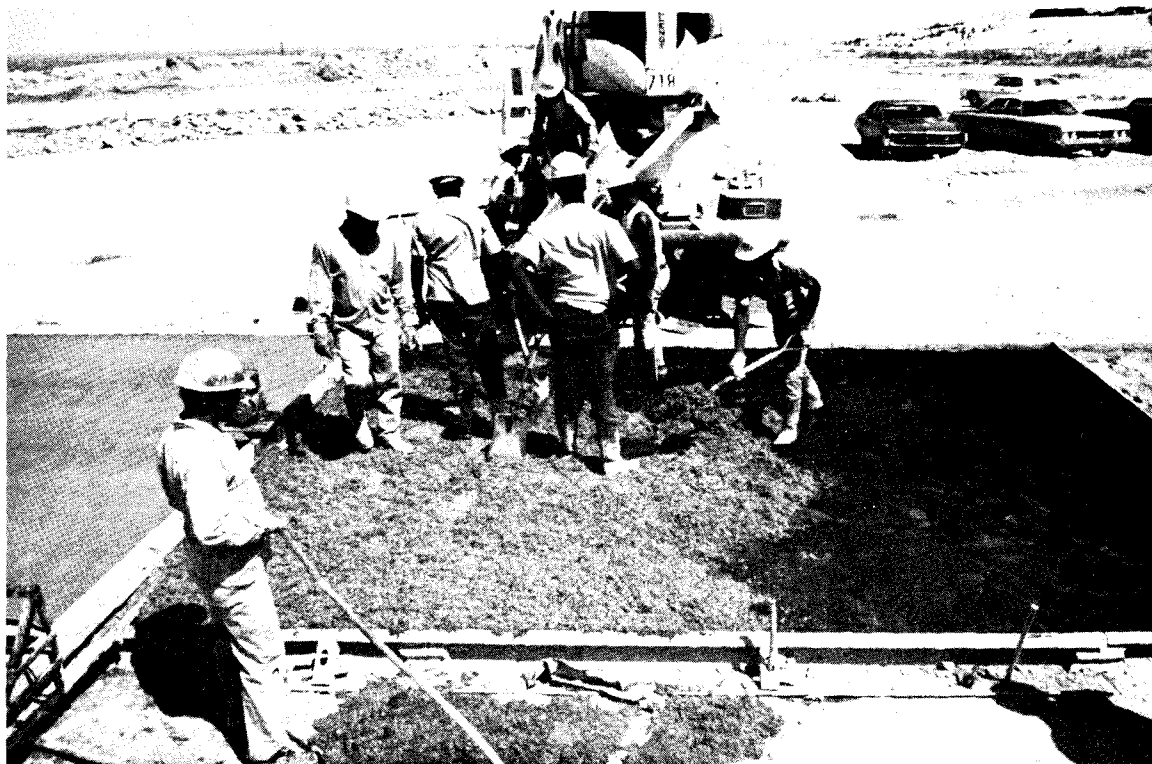
Figure 6: LOW SLUMP FIBER REINFORCED CONCRETE (AT \frac{V_r}{V} = 1.34\% ) REQUIRED EXTRA EFFORT IN PLACEMENT
