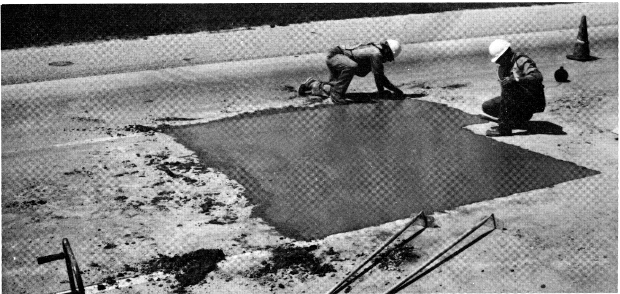
Figure 10: FINISHING OF PATCH #3
