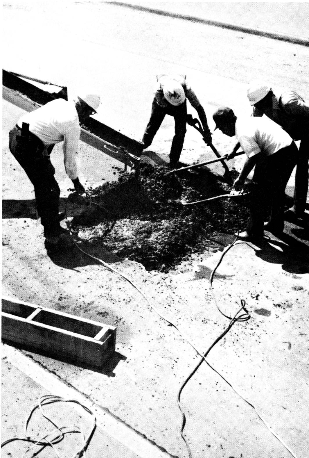
Figure 4: PLACING FIBER REINFORCED CONCRETE IN PATCH #1
