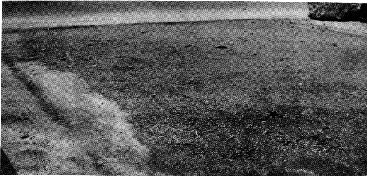
Figure 13: CLOSE UP SHOWING ABRASION OF PATCH #2
