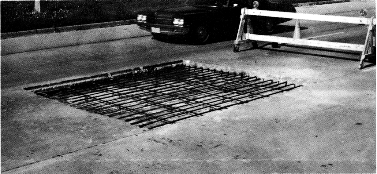
Figure 11: EXCACATION OF PATCH #4
