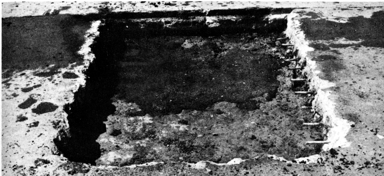
Figure 2: PATCH #1 BEFORE BEING FILLED WITH FIBERGLAS REINFORCED CONCRETE
