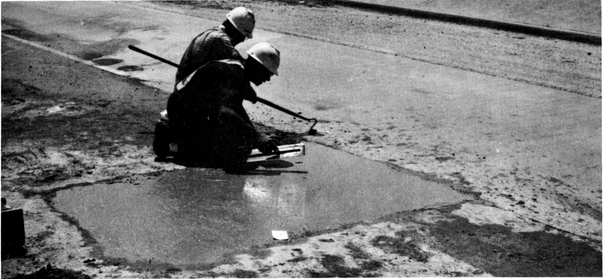
Figure 5: FINISHING OF CONCRETE IN PATCH #1
