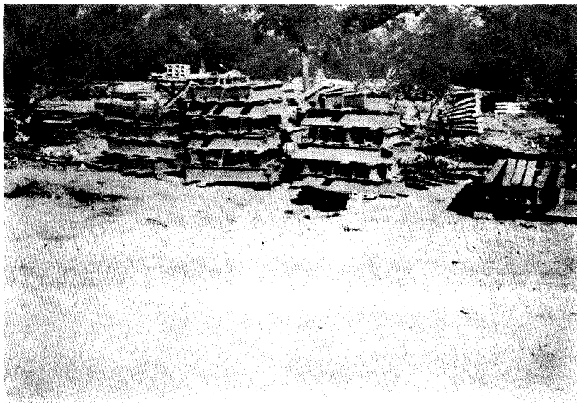
Salvaged I-beams from the old truss cut to lengths for guard rail posts to support proposed flex-beam railing.
