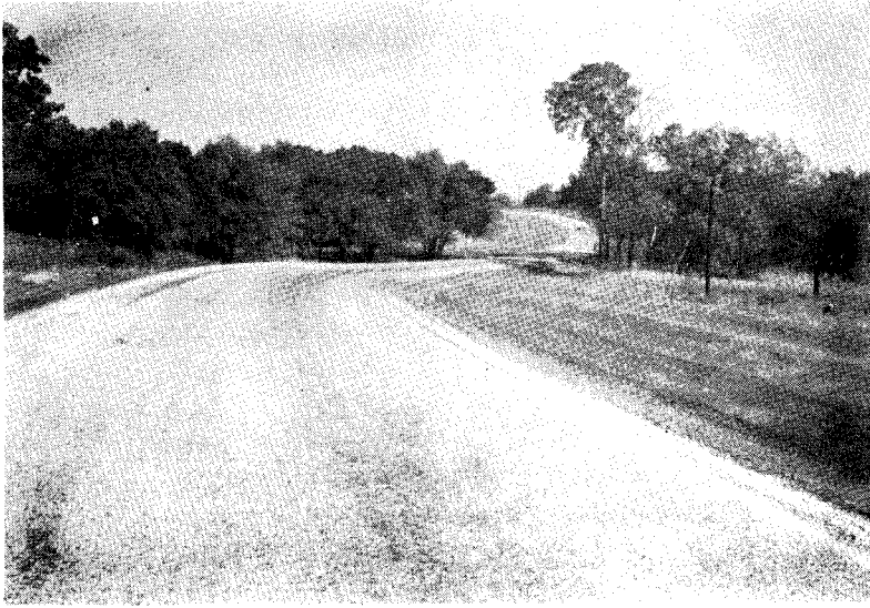
7 and 5 deg. curves well daylighted for sight distance. 100 ft. R.O.W., 18 ft. surface; 20 ft. finished crown, 26 ft. subgrade crown, usual 6:1 side slopes; "V" Type ditches - 24 ft. width structure in background used in place
