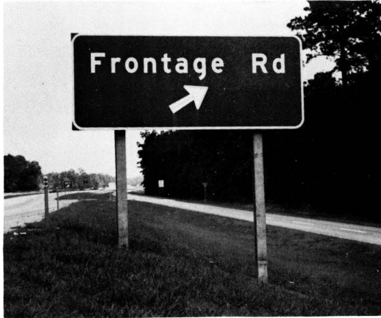
(a) View of break-away sign located on side slope.
