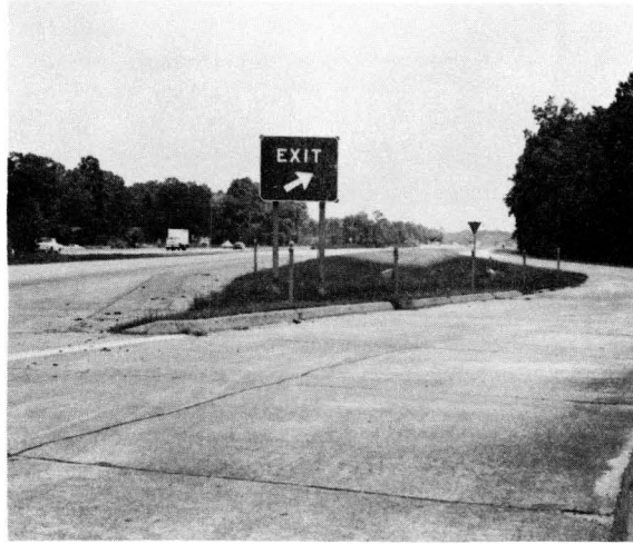
(a) View of break-away exit sign located in the gore.
