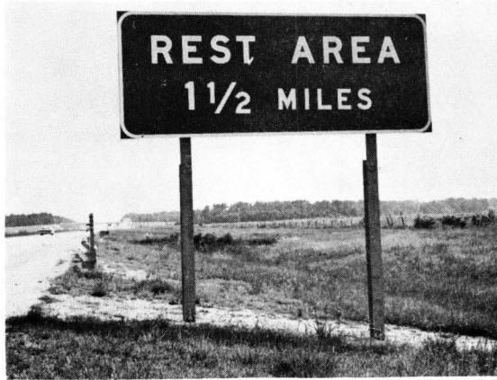
(a) Break-away roadside sign located near guardrail and bridge.
