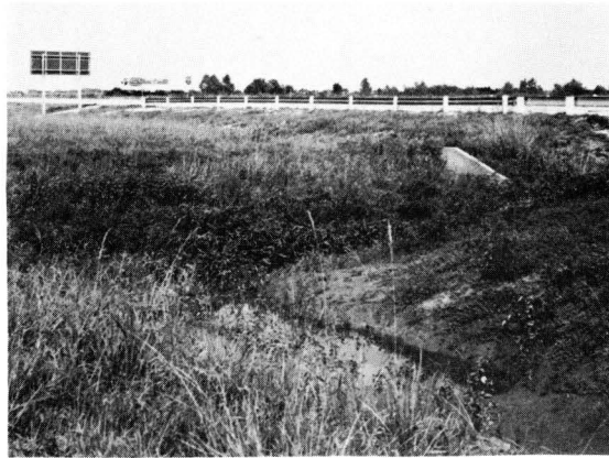
(b) Note relation of sign to guardrail, headwalls, and ditch.
