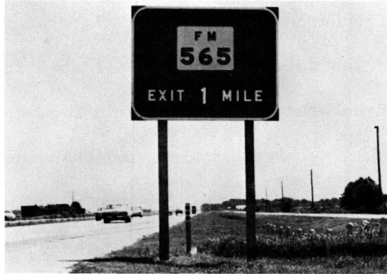
(a) View of break-away roadside sign located adjacent to shoulder.
