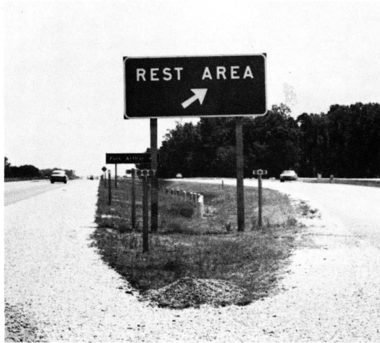
(a) Typical break-away rest area exit sign located in the gore.
