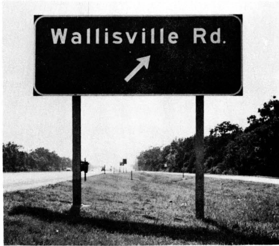
(a) Typical roadside break-away location.
