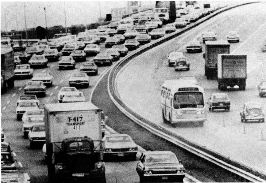
Boston, 1972 - bus operating in reserved lane of freeway in reverse direction during peak-hours.
