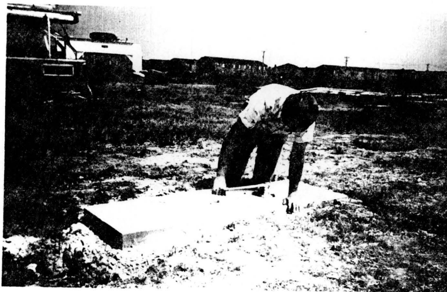
Figure 2 - SWECS Foundation
