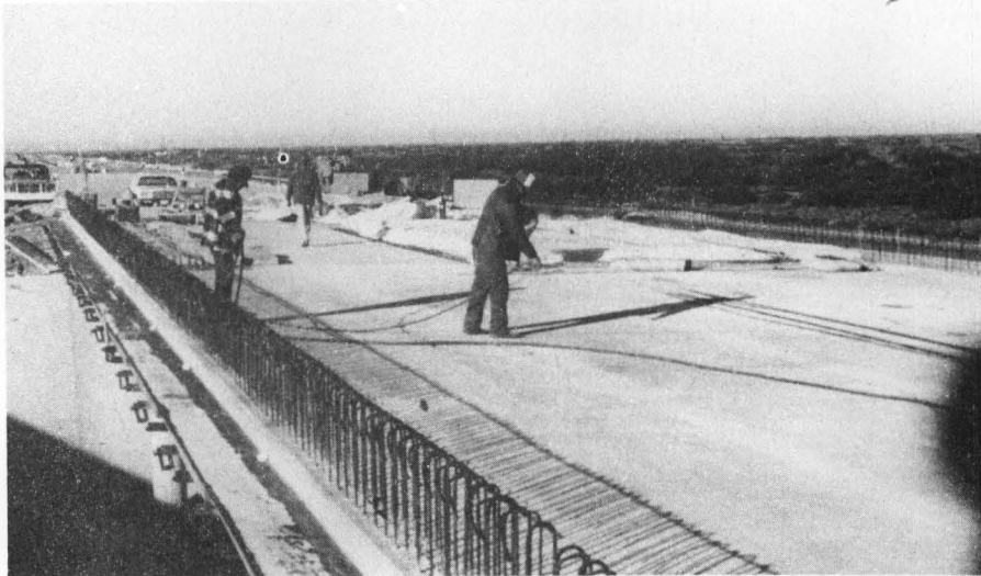
Figure 3. Cleaning Deck with Compressed Air
