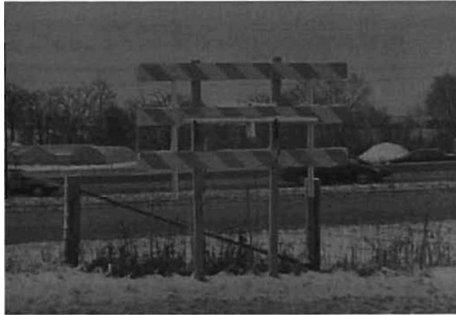
Figure 2-2 Type III Barricade Traffic Gate (Stored Position)
