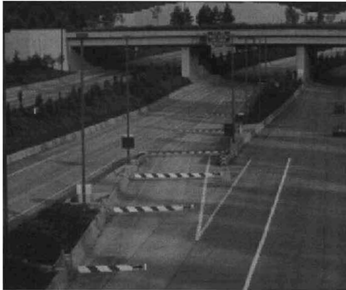
Figure 2-4 Horizontal swing gate( Chicago)
