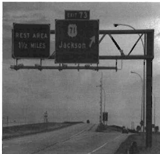
Figure 2-9 Minnesota IH-90 ramp closure gate
