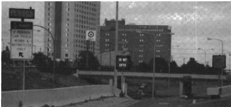
Figure 2-7 Variable ramp closure using signing in St. Paul, Minnesota
