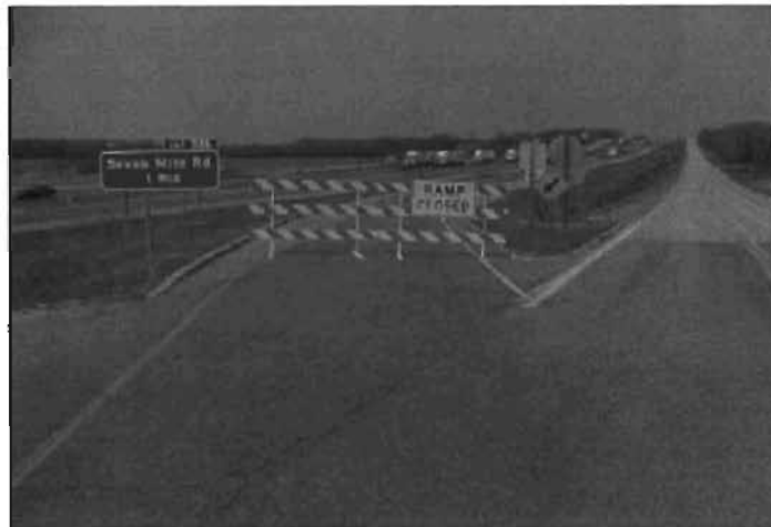
Figure 2-3 Type III Barricade Traffic Gate (Deployed)
