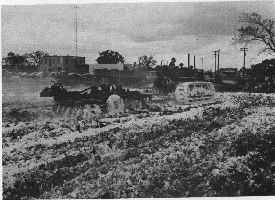
Photograph No. 14 Showing mixing operations.
