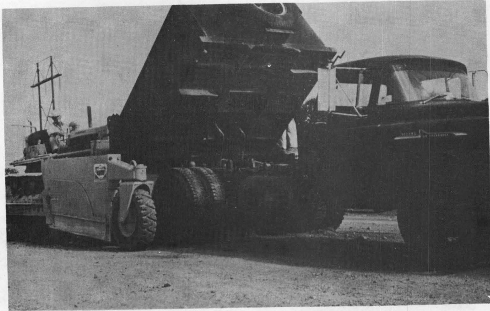
Photograph No. 18, showing final mix being end dumped into spreader box.
