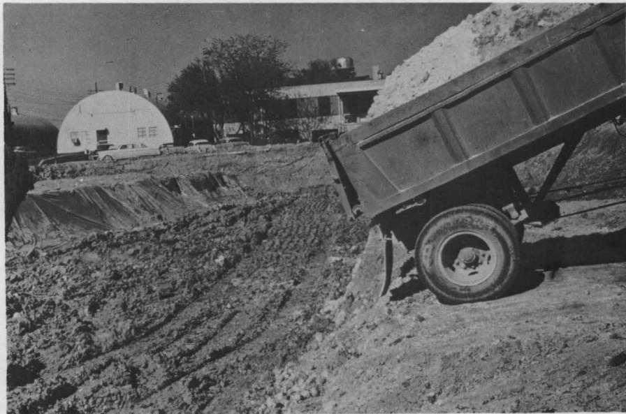
Photograph No. 6 Dumping of lime on subgrade.
