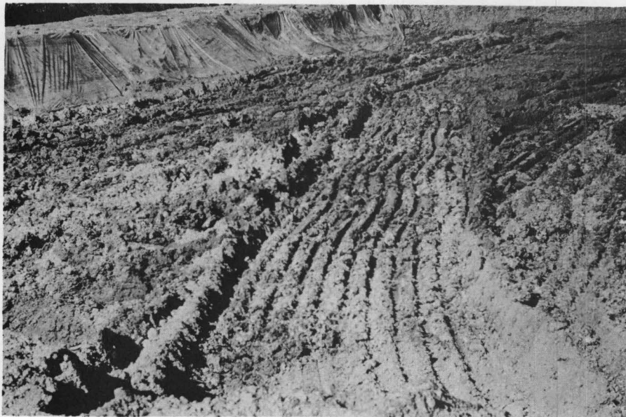
Photograph No. 8 Same as Photograph No. 7, showing streaks left by teeth of front end loader bucket.
