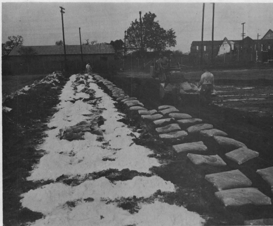
Photograph No. 13 Showing application of lime.
