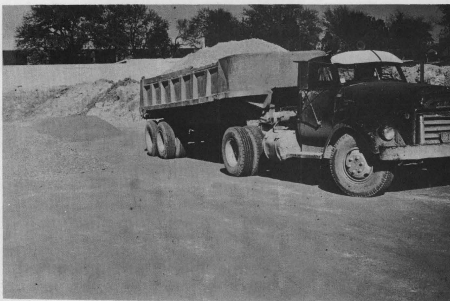
Photograph No. 10 Lime-treated subgrade supports heavy loads of base material only 3 days after adding lime to very soft clay subgrade.
