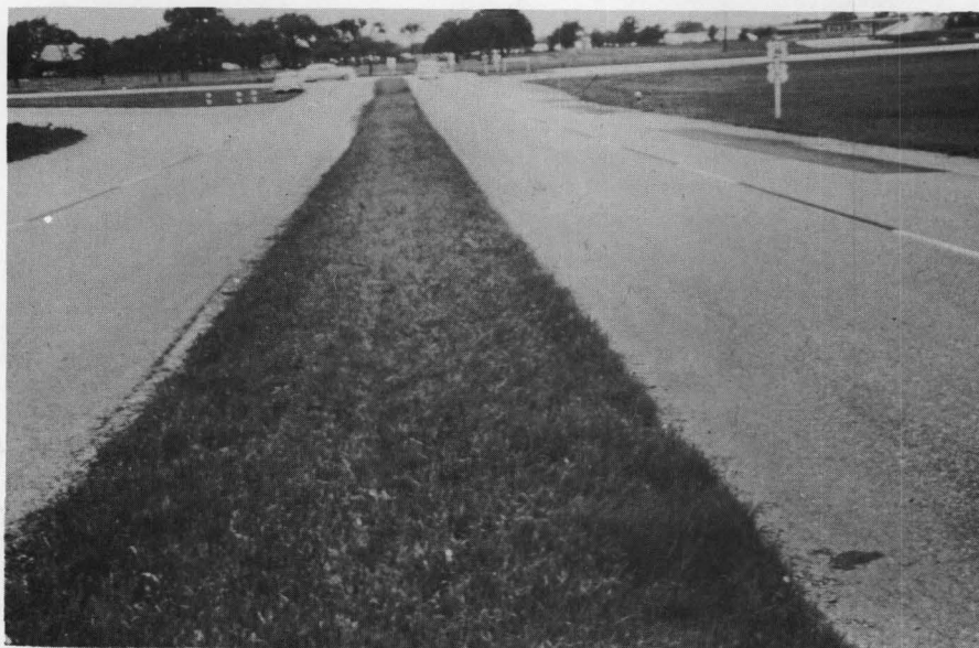
Photograph 3, taken 6 years later at same location as Photograph 1. Note patches on untreated section at right and excellent condition of treated section at left after 14 years of service.
