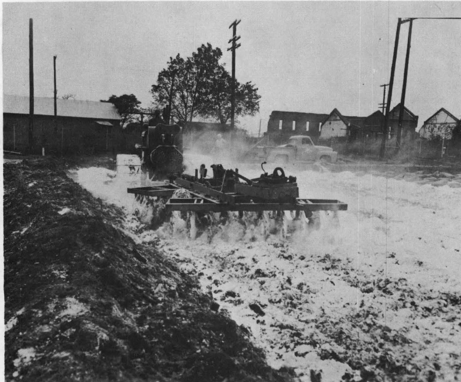
Photograph No. 15 Showing mixing operations.
