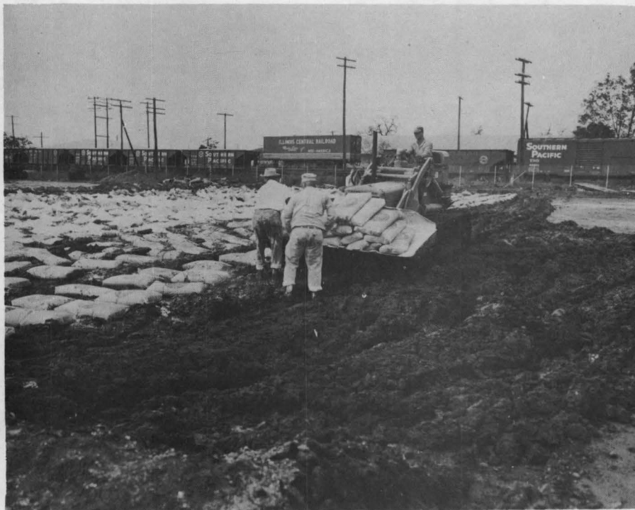
Photograph No. 12 Showing application of lime.
