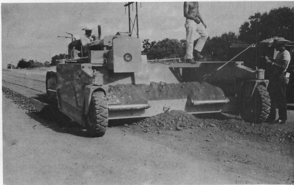
Photograph No. 19, showing the Blaw-Knox Spreader Box.
