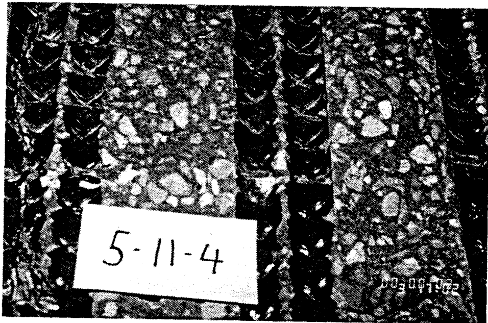
Figure 3.3 Cover on Coated Bars After Test
