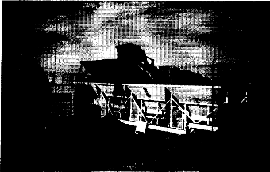
Figure 4.19. Combined new and reclaimed material cold feed bins
