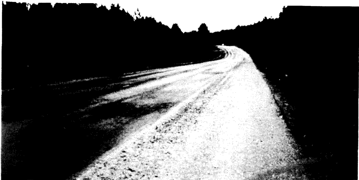
Figure 11.4. Systematic spot segregation between truckloads
