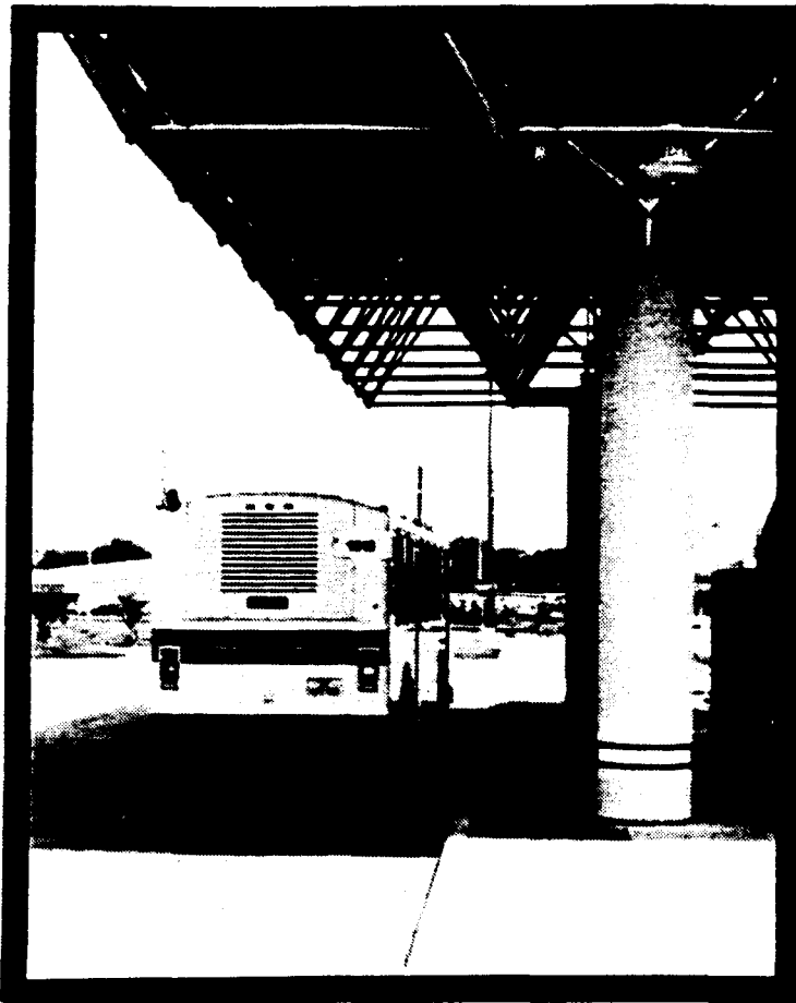
Figure 35 : Bus Awning at Capital Metro Park-and-Ride Facility: U.S. 183 and Lamar Blvd.
