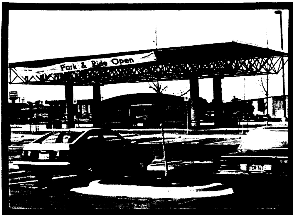
Figure 36 : Bus Passenger Shelter at Capital Metro Park-and-Ride Facility: U.S. 183 and Lamar Blvd.
