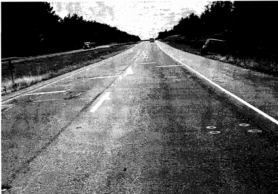
Figure 2.1 Southbound view of US 59 at north site
