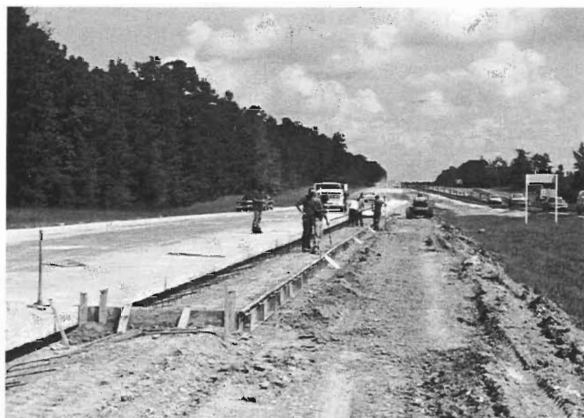
Figure 3.8. Excavation and preparation for shoulder extension
