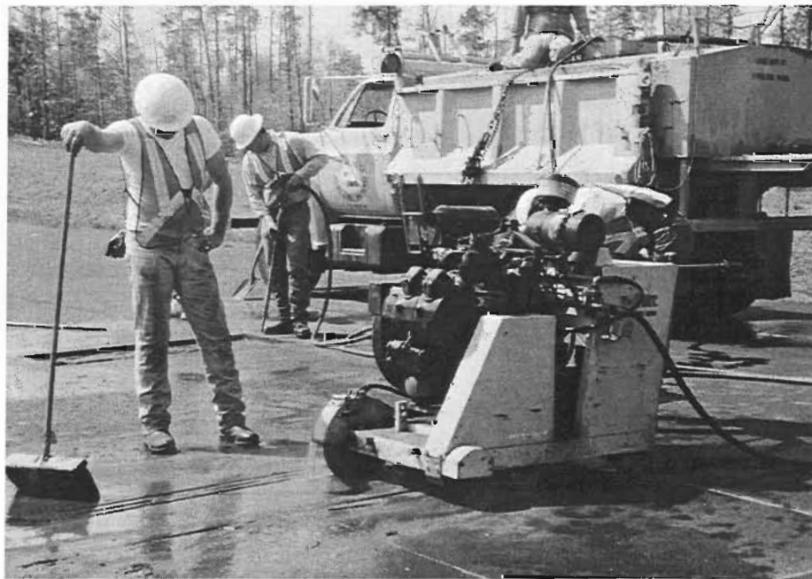
Figure 5.2. Concrete saw used to remove overlay at WIM site
