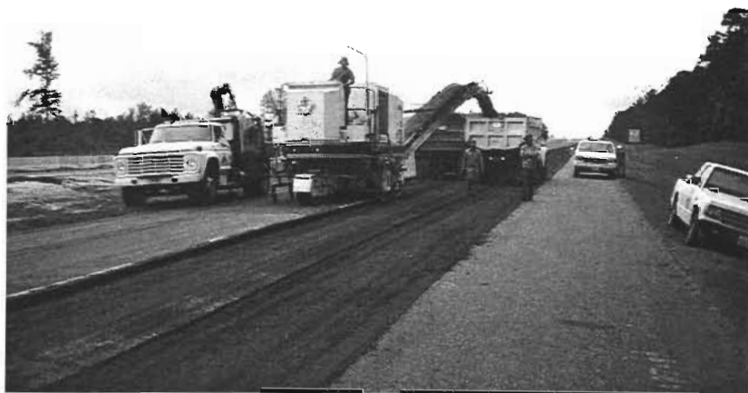
Figure 3.13. Roto-milling of Section R2
