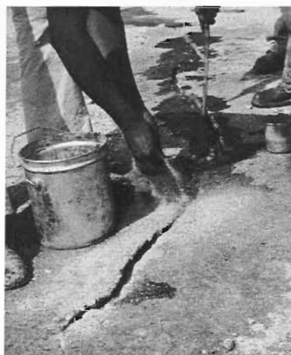
Figure 3.6. Placement of HMWM and sand
