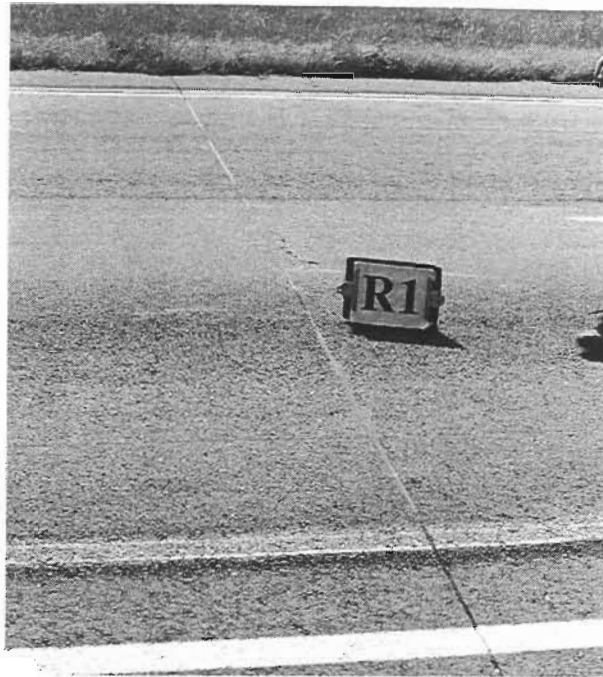
Figure 3.11. Saw cut over joint in R1
