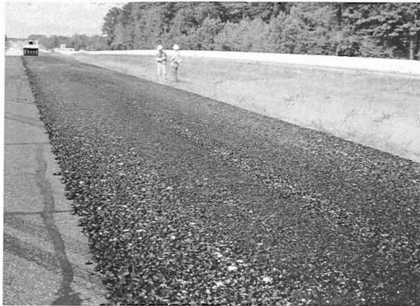
Figure 3.20. Placement of Type G material in R4
