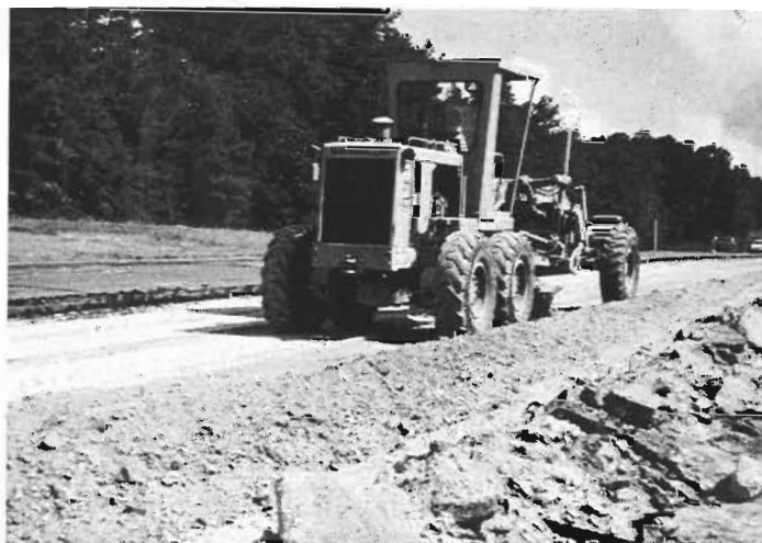
Figure 3.2. Blading of fill material for preparation of base
