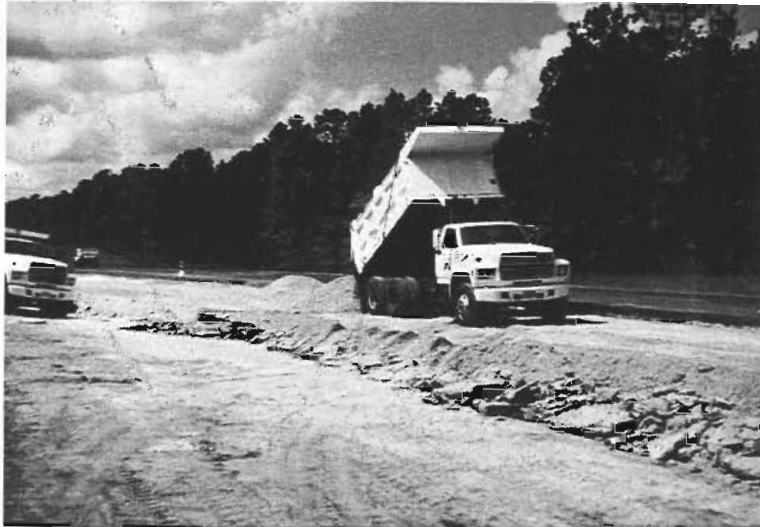
Figure 3.1. Hauling of fill material to Detour #4
