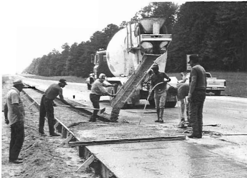
Figure 3.10. Placement of extended shoulder
