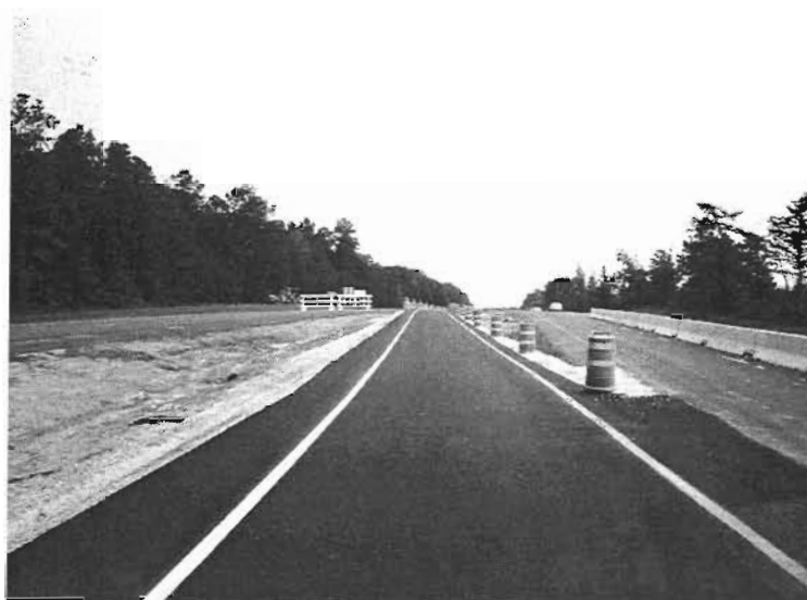
Figure 3.3. Finished view of Detour #4
