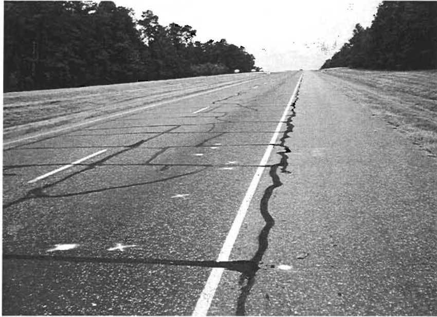
Figure 2.3. Rigid sections prior to rehabilitation
