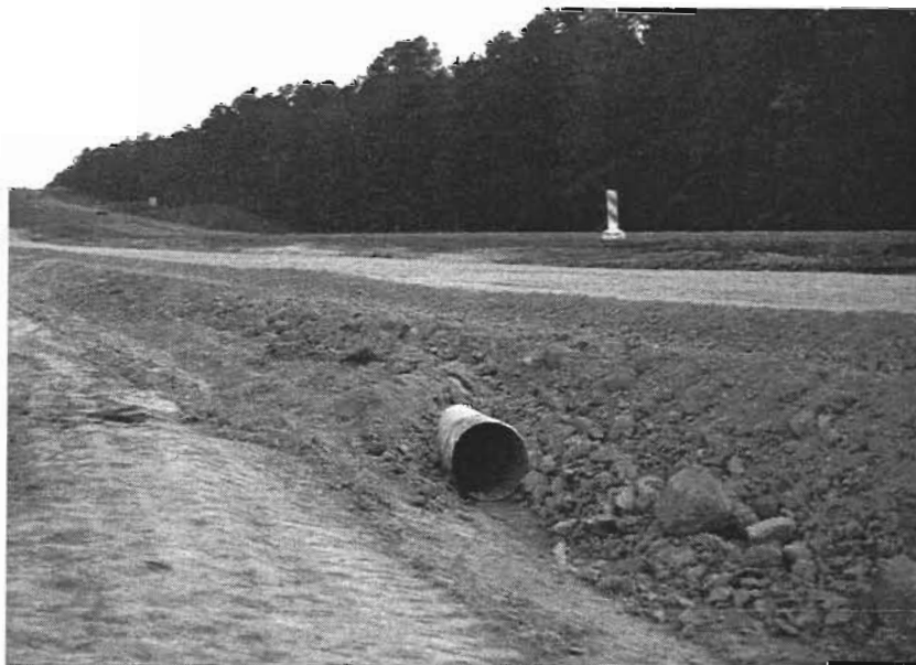
Figure 4.2. Pipe placement in Detour #2
