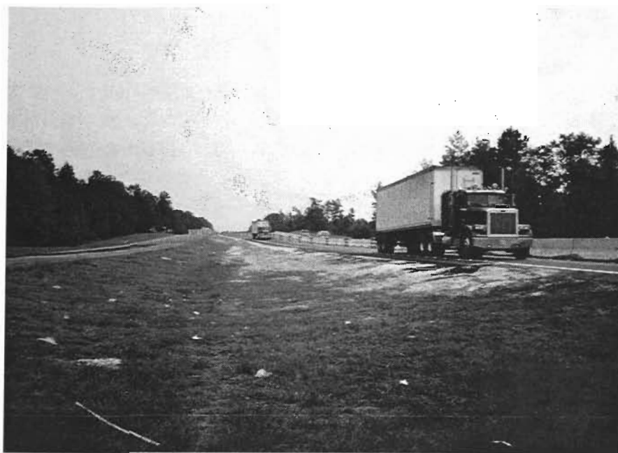
Figure 4.3. Failing detour under traffic
