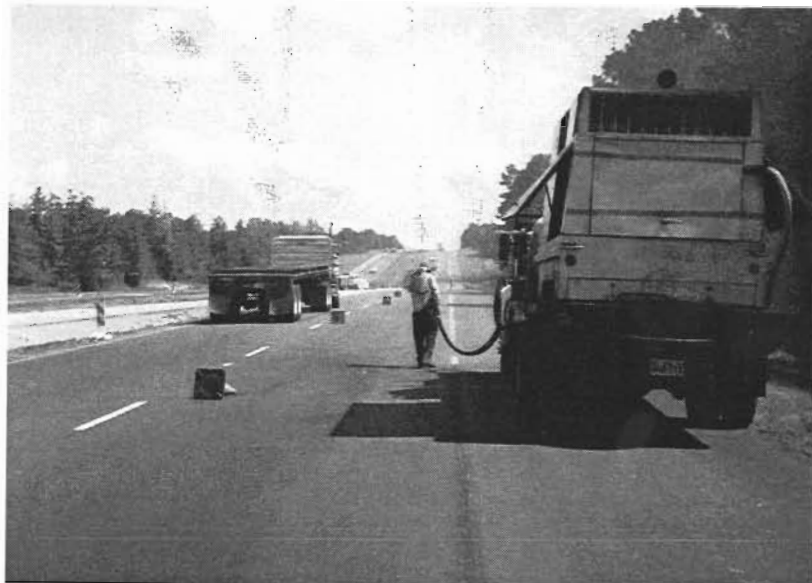
Figure 3.25. Sandblaster removing striping
