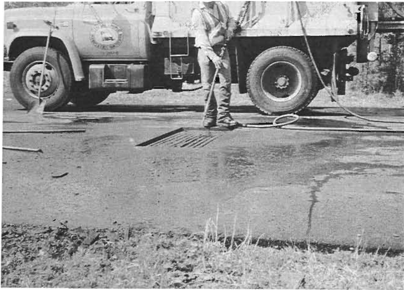
Figure 5.3. Sandblaster preparing WIM pad site
