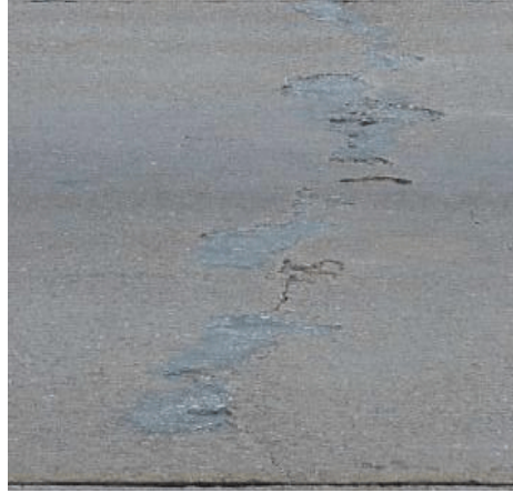
Crack Spalling
