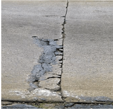
Joint Failure
