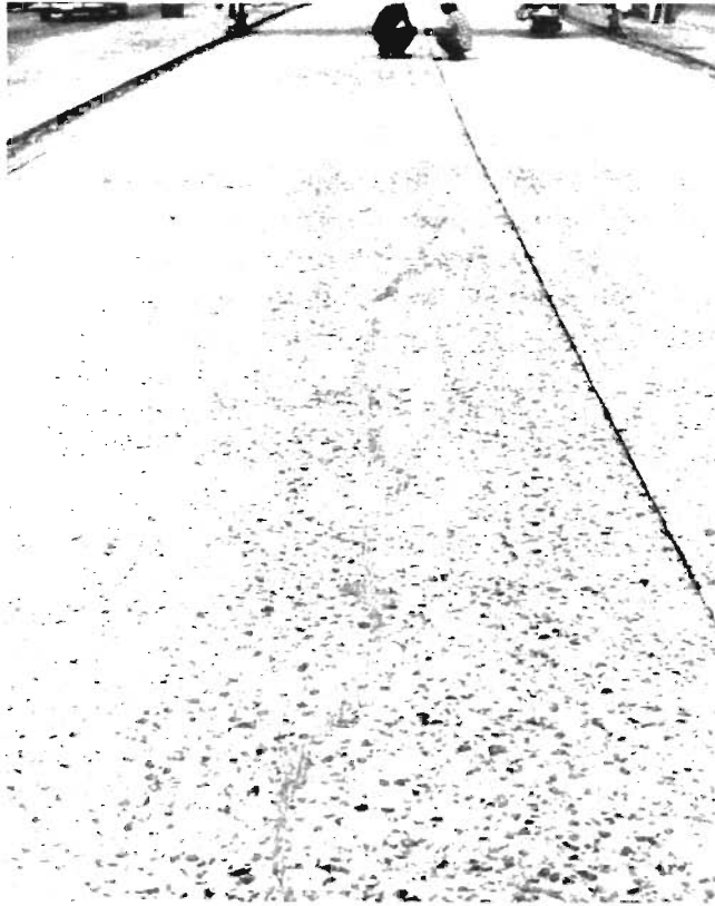
Longitudinal cracking on IH-610 test section after crack filling and milling, before construction of thin bonded overlay.
