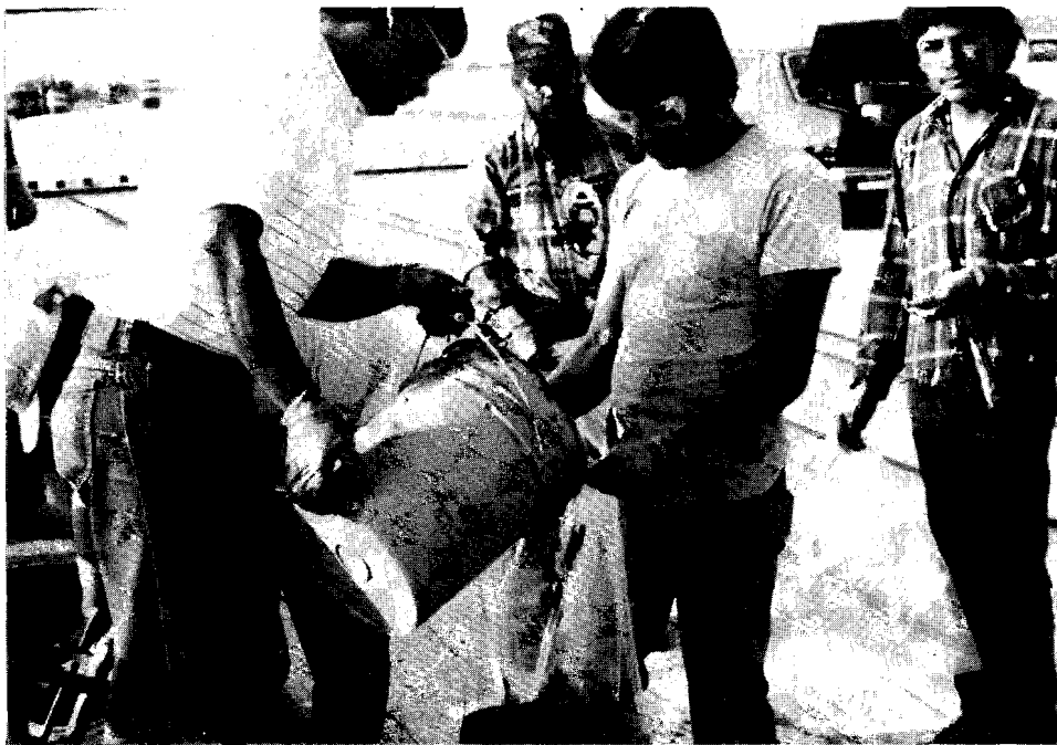
Figure III.18 System "C" Transfer of mixture to placement bags
