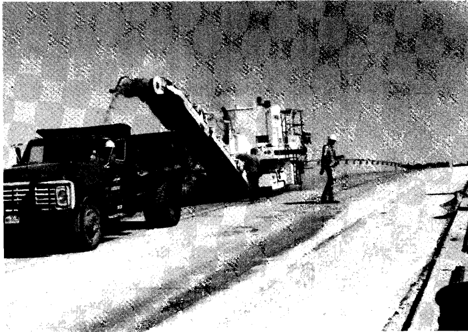
Figure III.1 U.S. 87 Overpass, milling operation by the contractor
