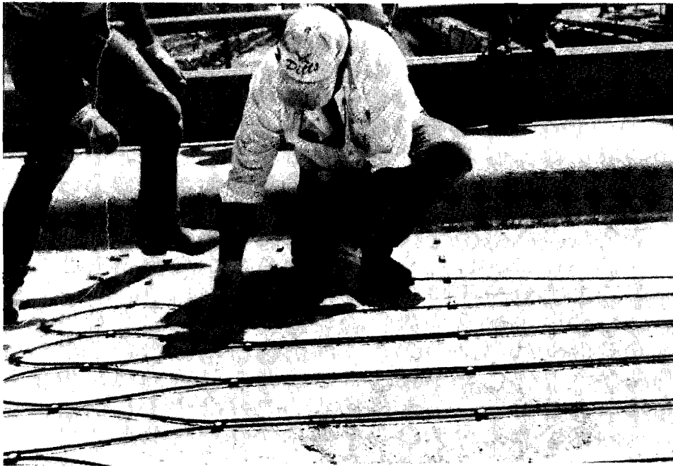
Figure III.14 System "B" installation of conduit
