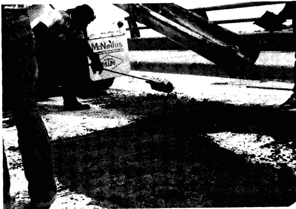
Figure III.5 Placement of concrete repair
