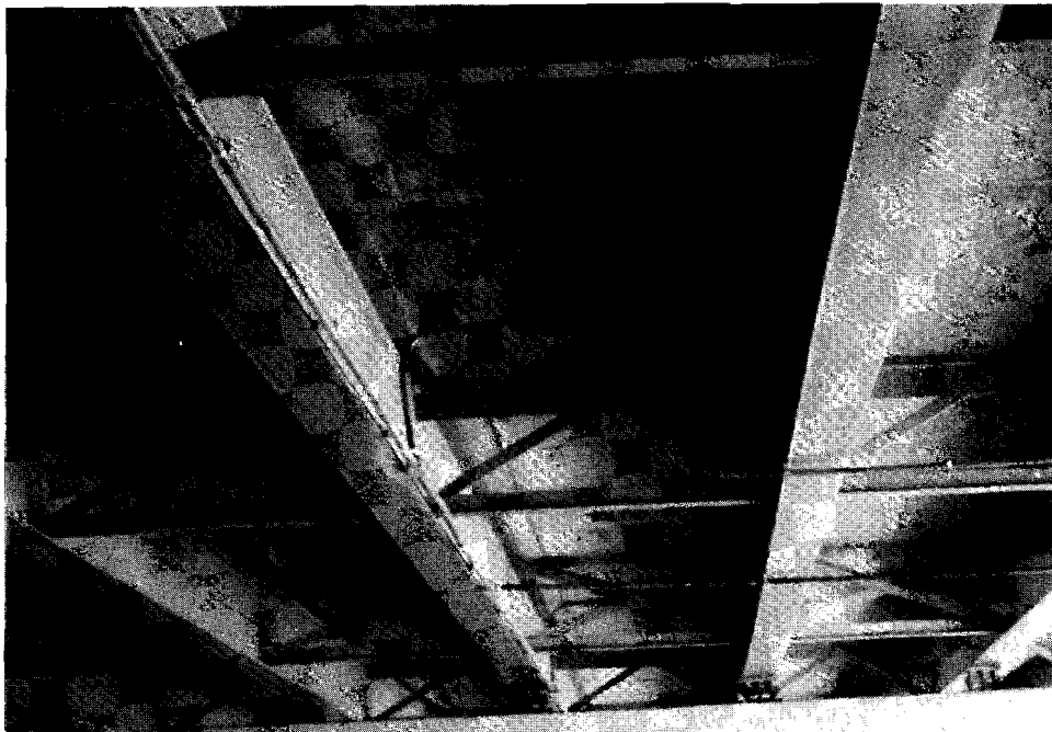
Figure III.29 Conduit runs under the structure
