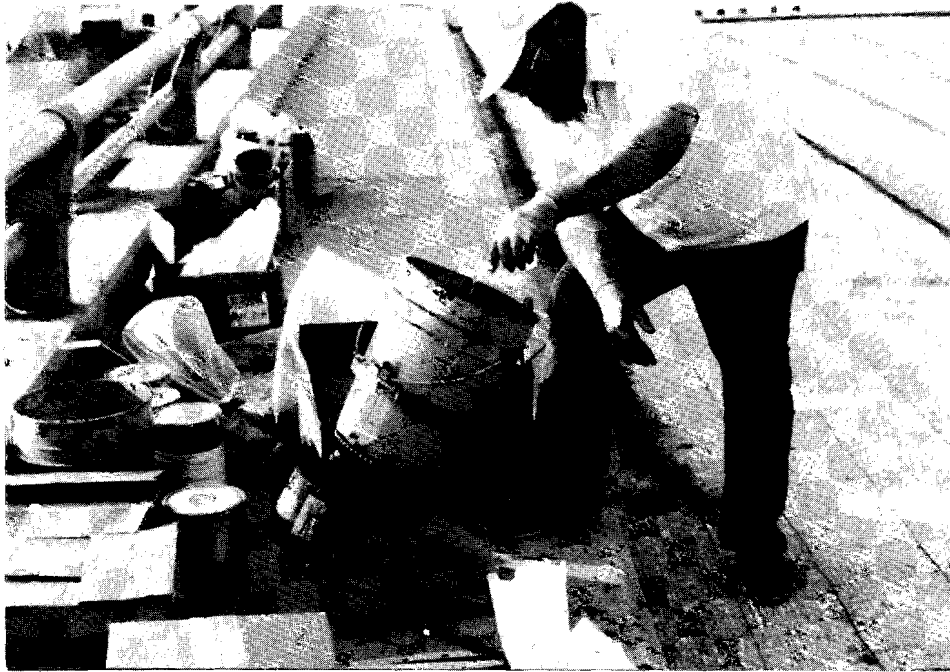
Figure III.17 System "C" Preparation of carbon mixture
