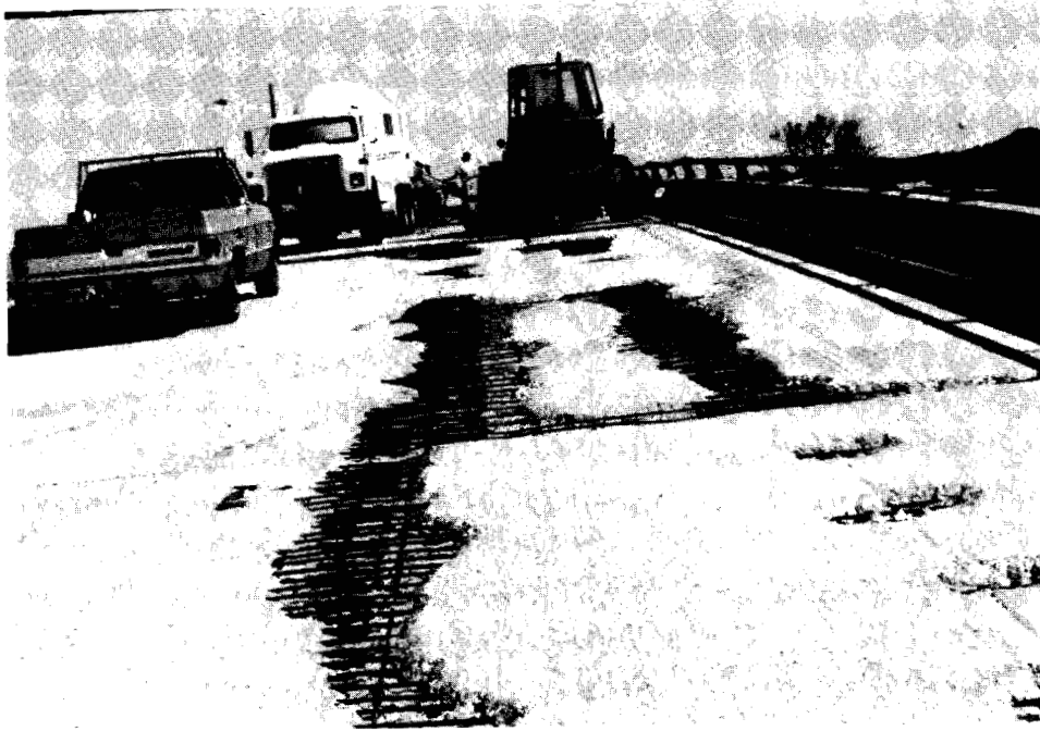
Figure III.4 Bridge deck prepared for placement of concrete repair
