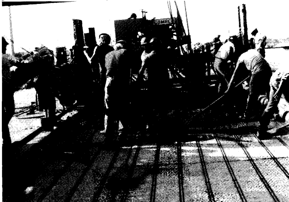
Figure III.16 System "B" Placement of dense concrete overlay
