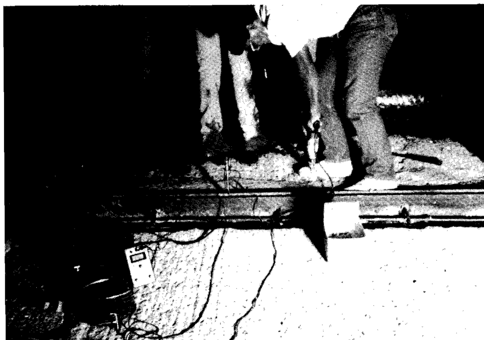
Figure III.12 Repair of System "A" short-out
