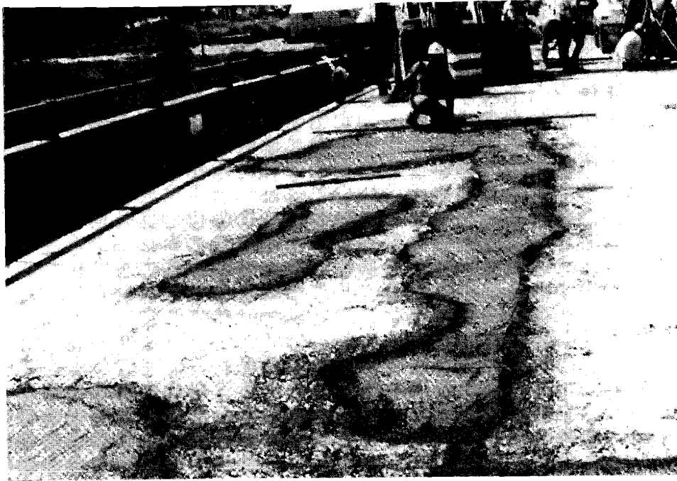
Figure III.6 Completed concrete deck repair
