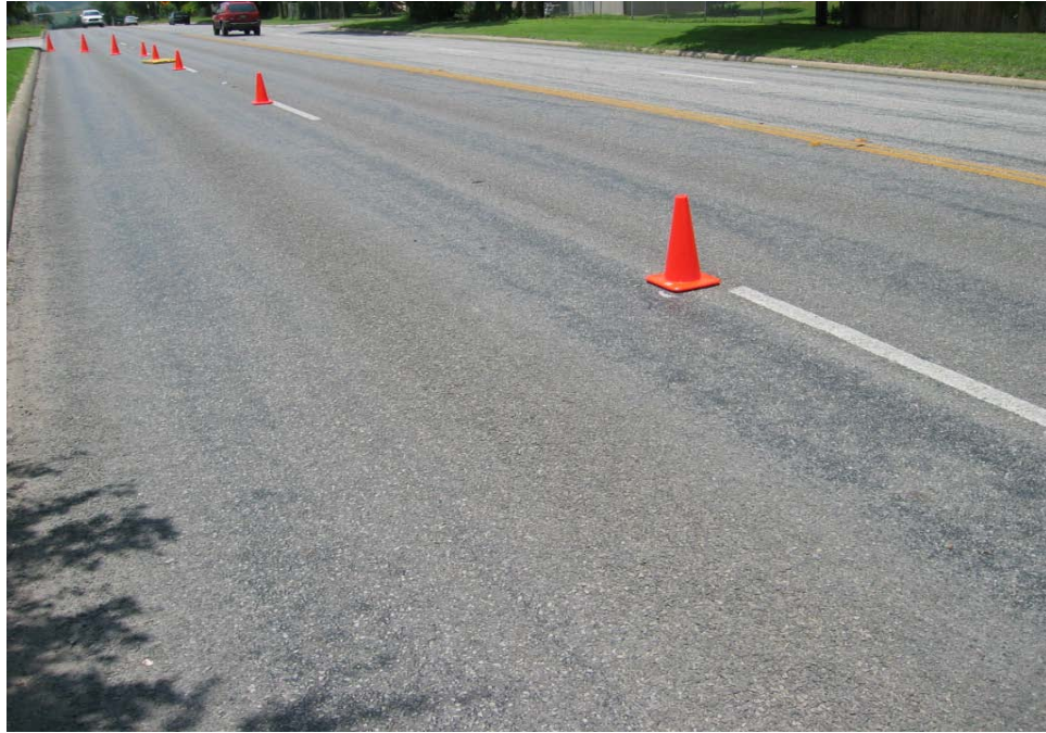
Figure A.5 Seal coat with moderate flushing
