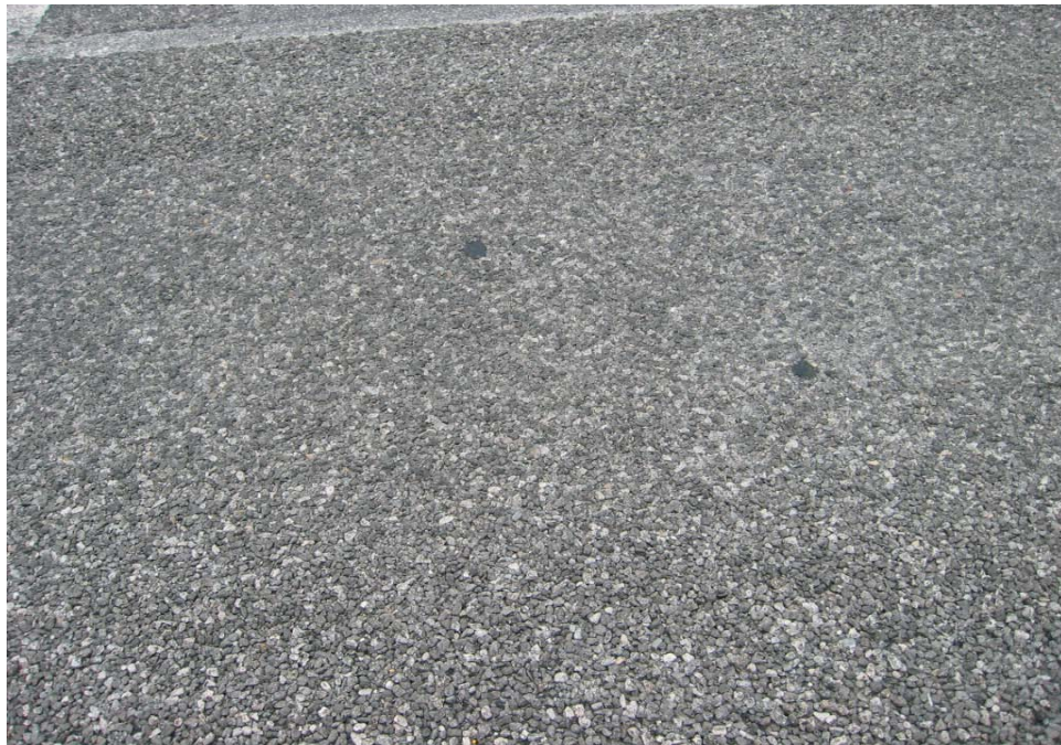
Figure A.2 New seal coat close up
