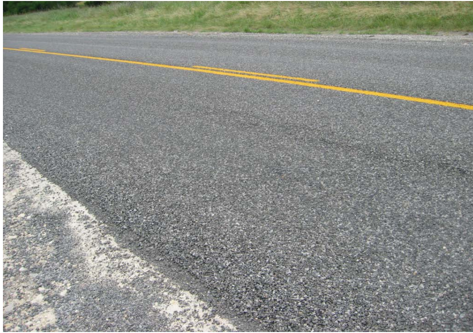
Figure A.1 New seal coat
