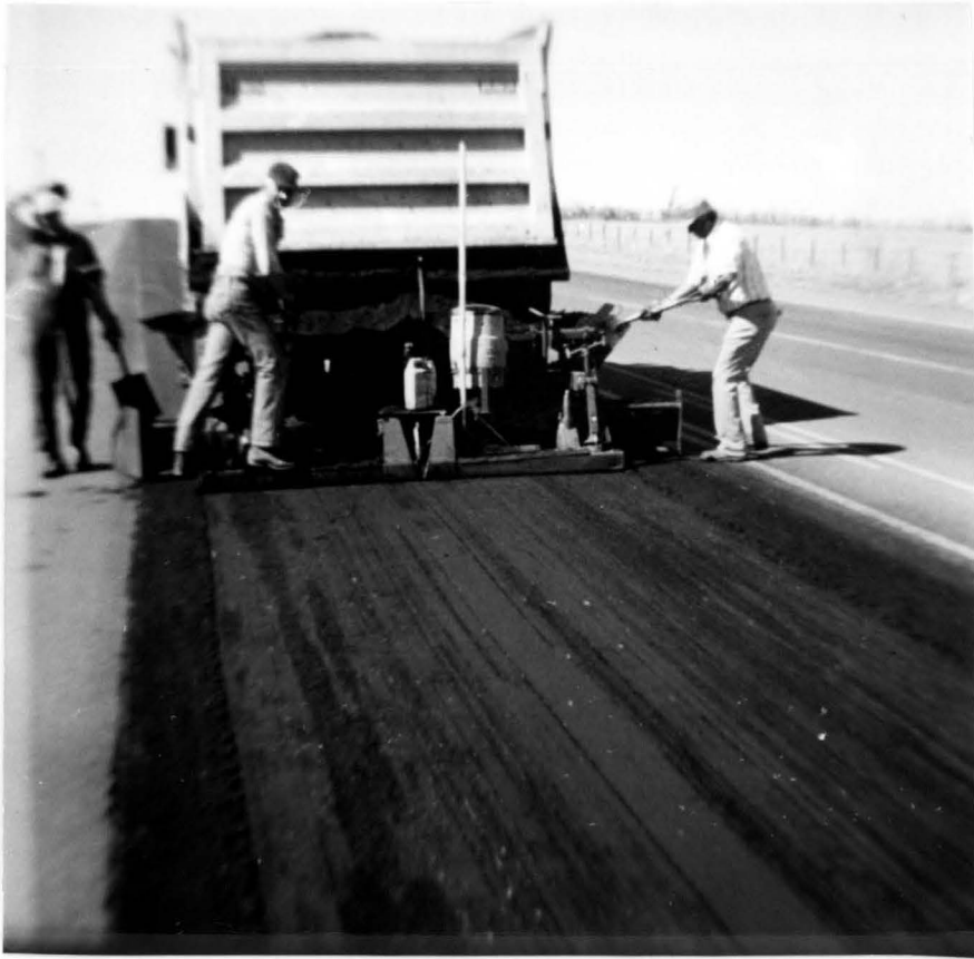
Sand asphalt mixture as it comes out drag box.
