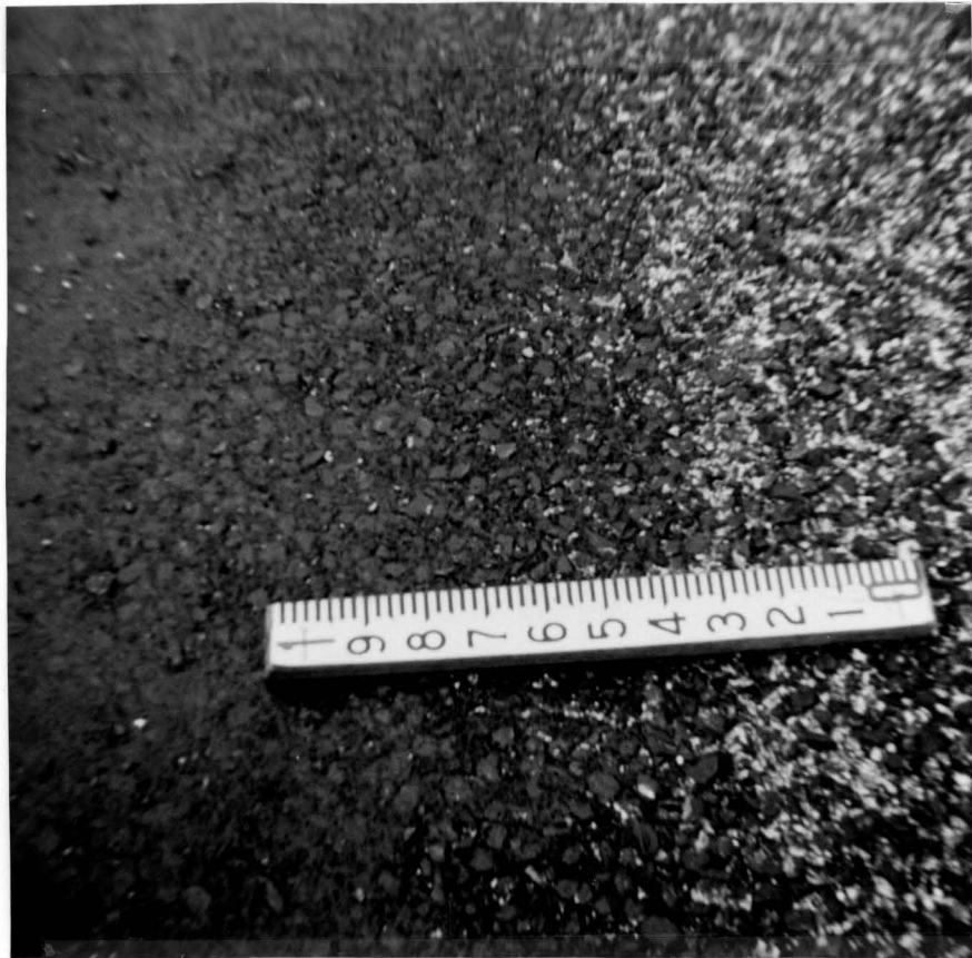
Traffic pressed seal coat aggregate into sand asphalt mix with flushing resulting.
