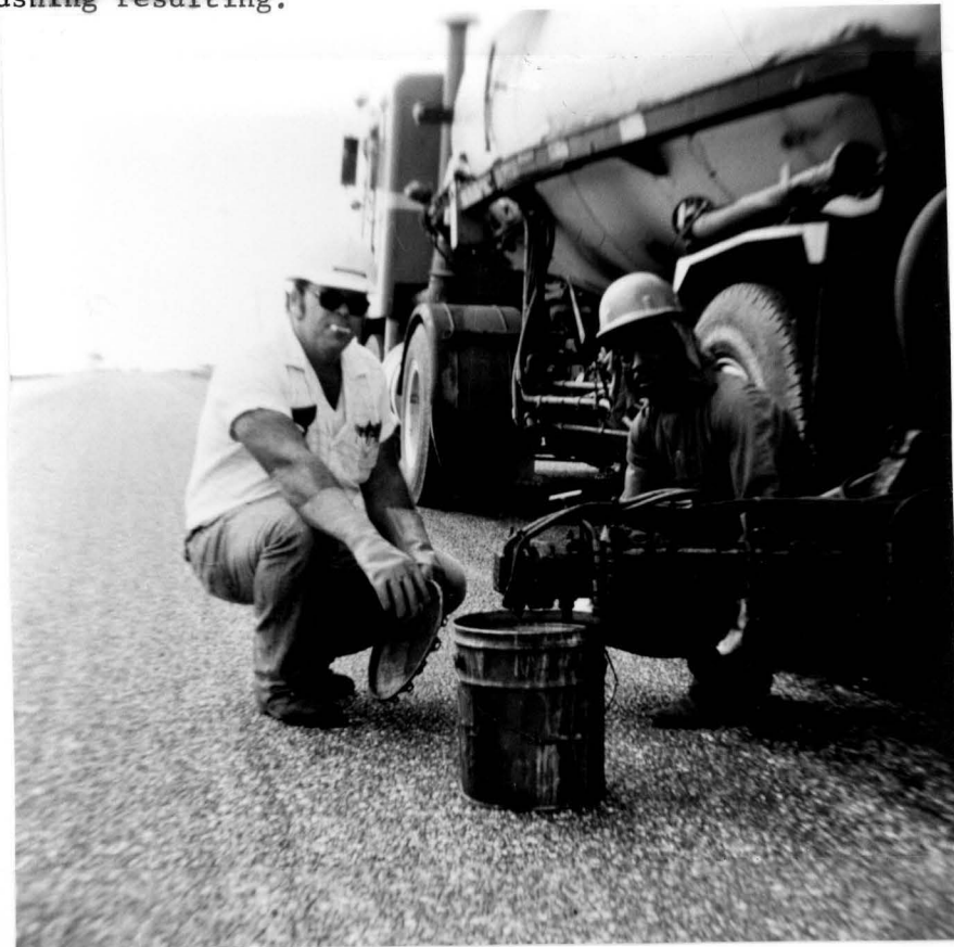
Traffic pressed seal coat aggregate into sand asphalt mix with flushing resulting.
