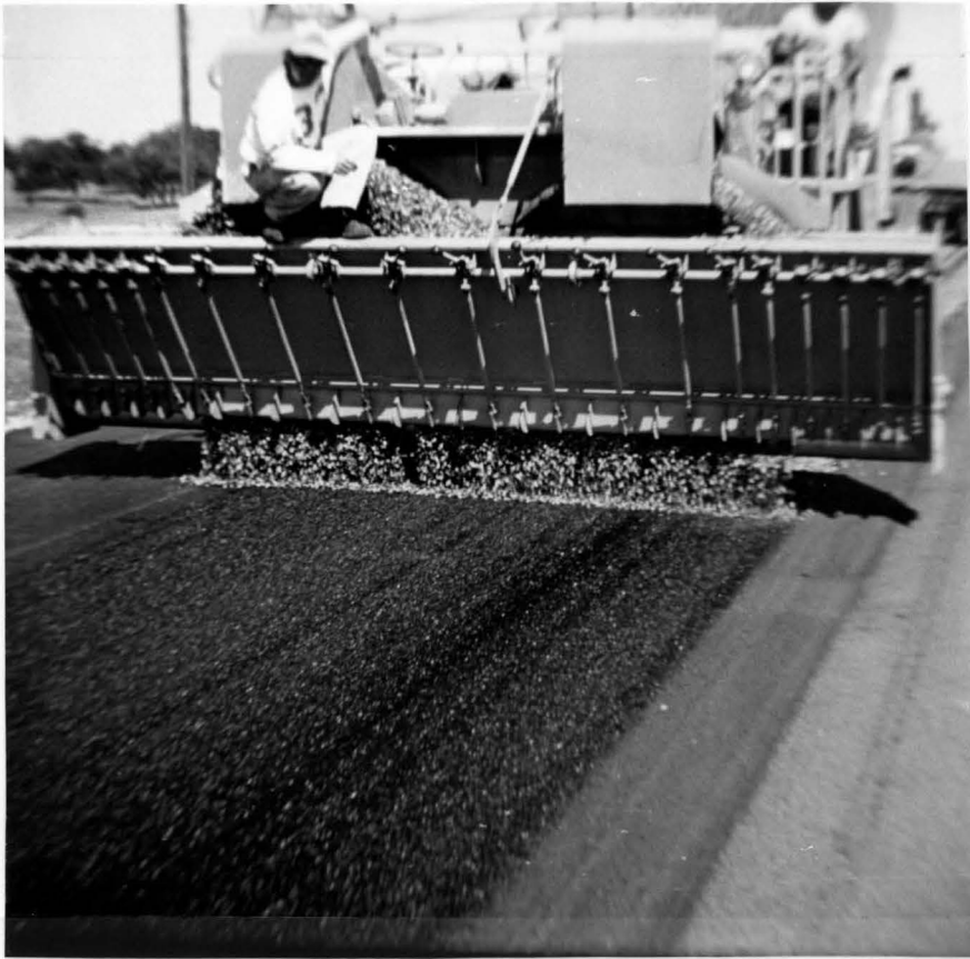
Bomag aggregate spreader.
