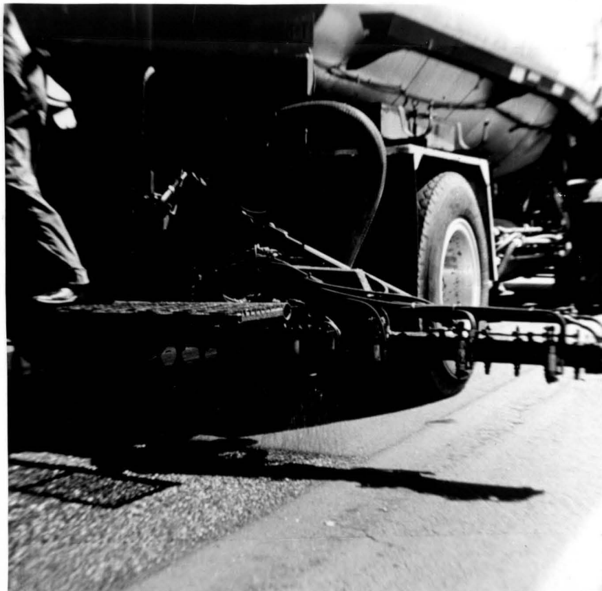
Application of asphalt-rubber seal coat using some nozzels.
