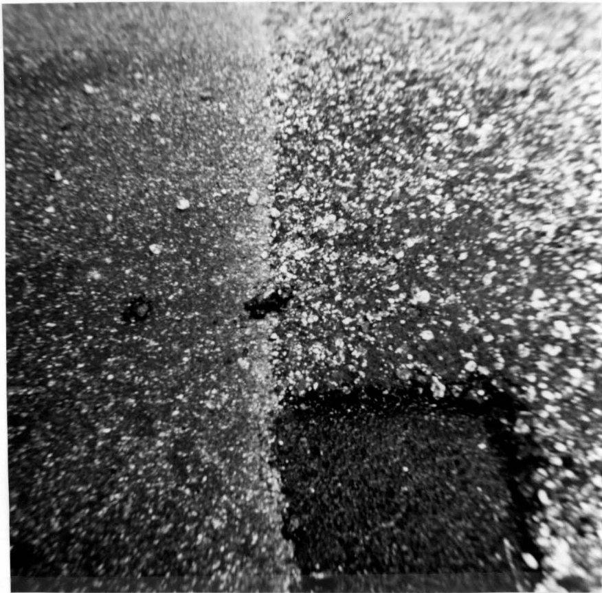
Cut out section shows thickness of asphalt-rubber seal coat.
