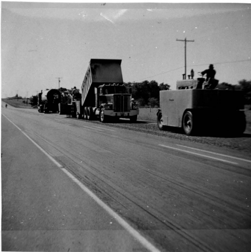
Bomag aggregate spreader.
