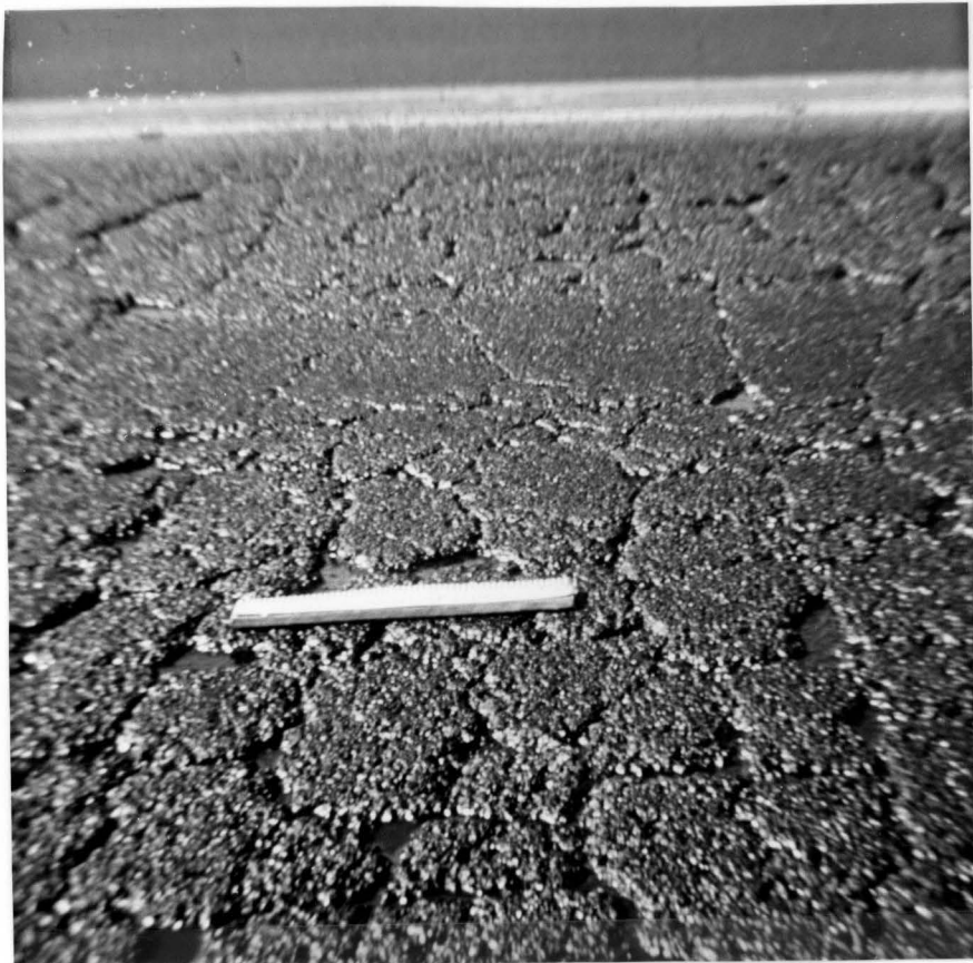
Heavily primed existing pavement prior to applying sand asphalt mix.
