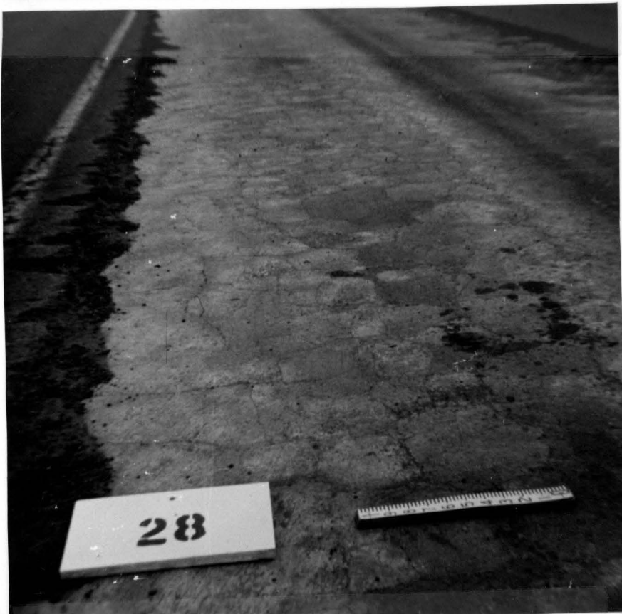
Old Slag aggregate hot mix cleaned and ready to prime.
