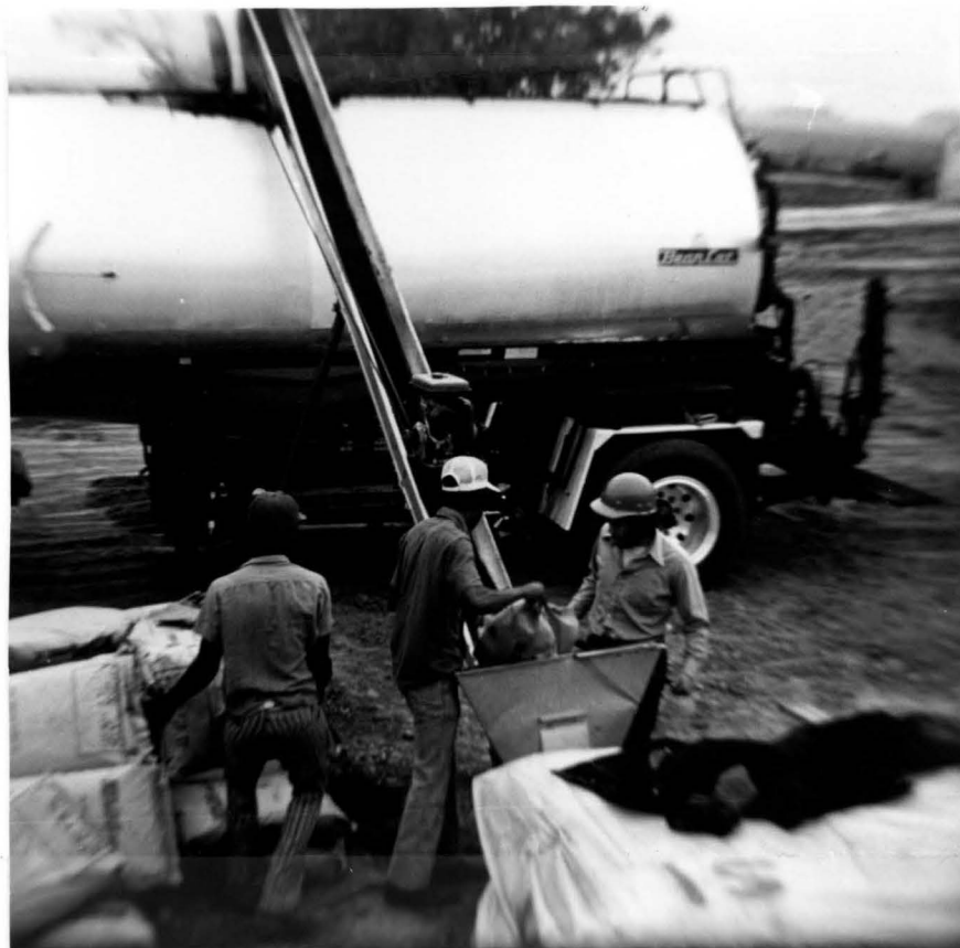
Ground rubber from ATLOS Rubber, Los Angeles, California, being carried on agricultural conveyor belt into distributor.
