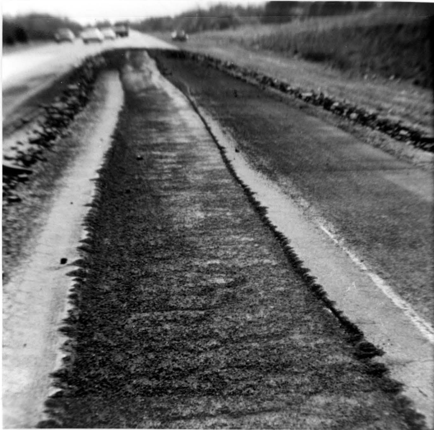
Rubber tired front end loader removing old lightweight aggregate hot mix that was no longer bonded to slag aggregate layer.
