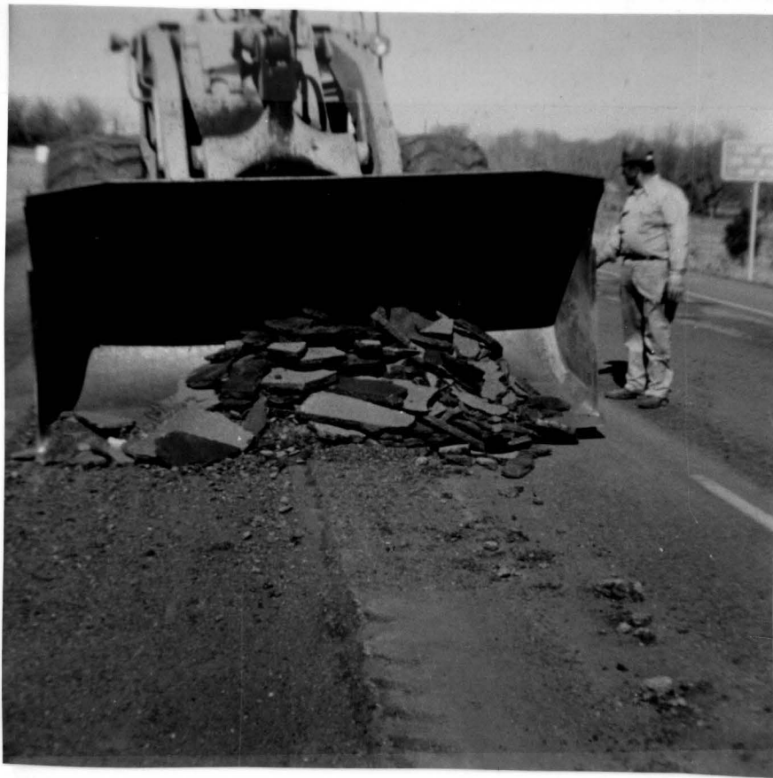
Rubber tired front end loader removing old lightweight aggregate hot mix that was no longer bonded to slag aggregate layer.
