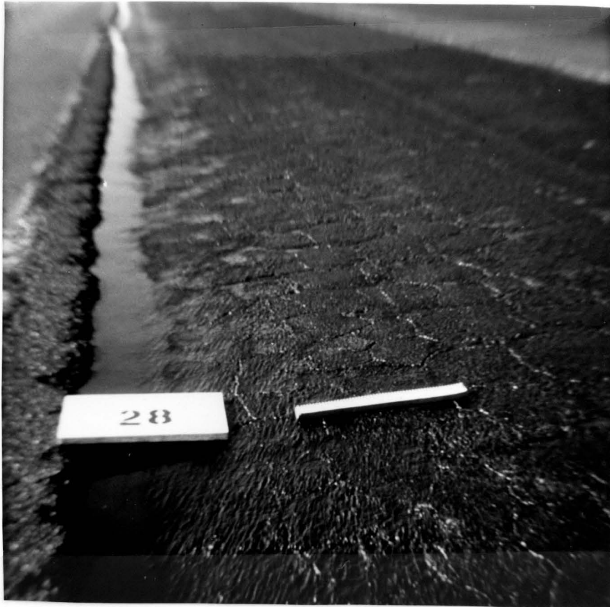
Old Slag aggregate hot mix cleaned and ready to prime.
