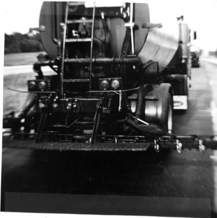
Rear view of Bear Cat distributor and spray bar.
