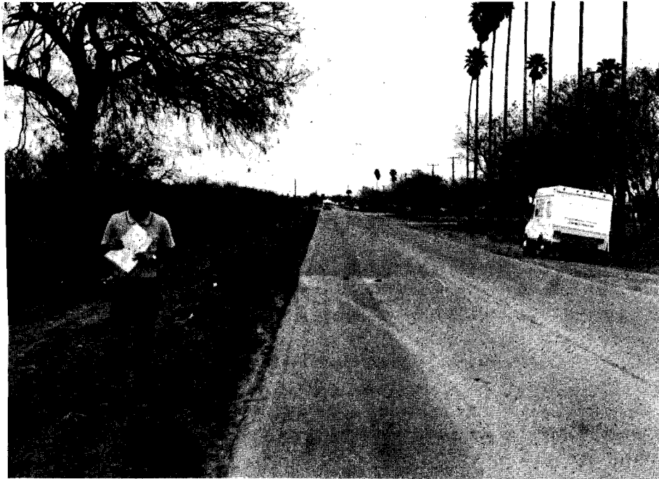
Photo taken in February of 1980 on the recycled pavement, used as a surface overlay, after 44 months of service.
