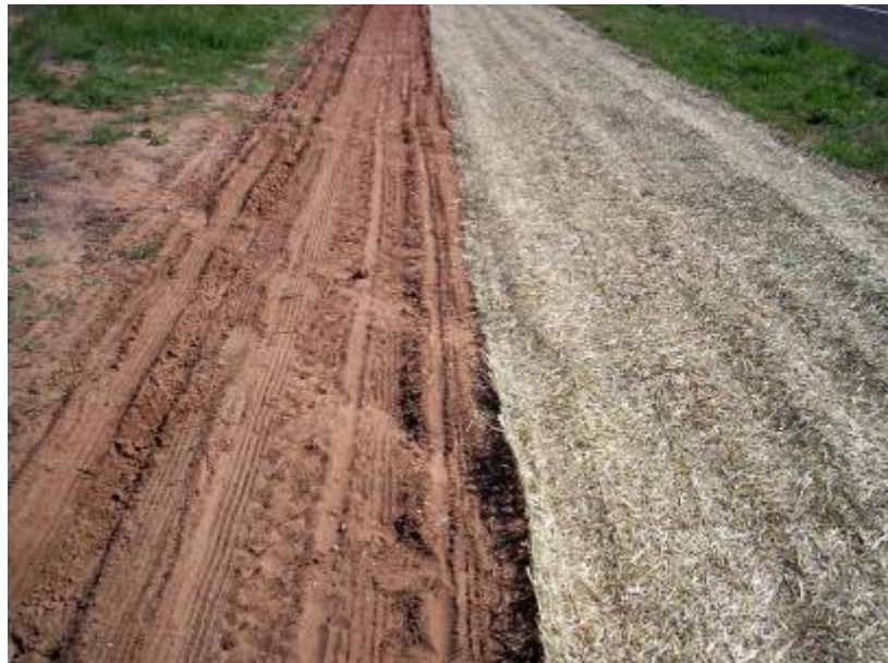
Figure 3-10. Single net straw blanket (S75BN™) from North American Green© in Andrews County, Texas, 2006.
