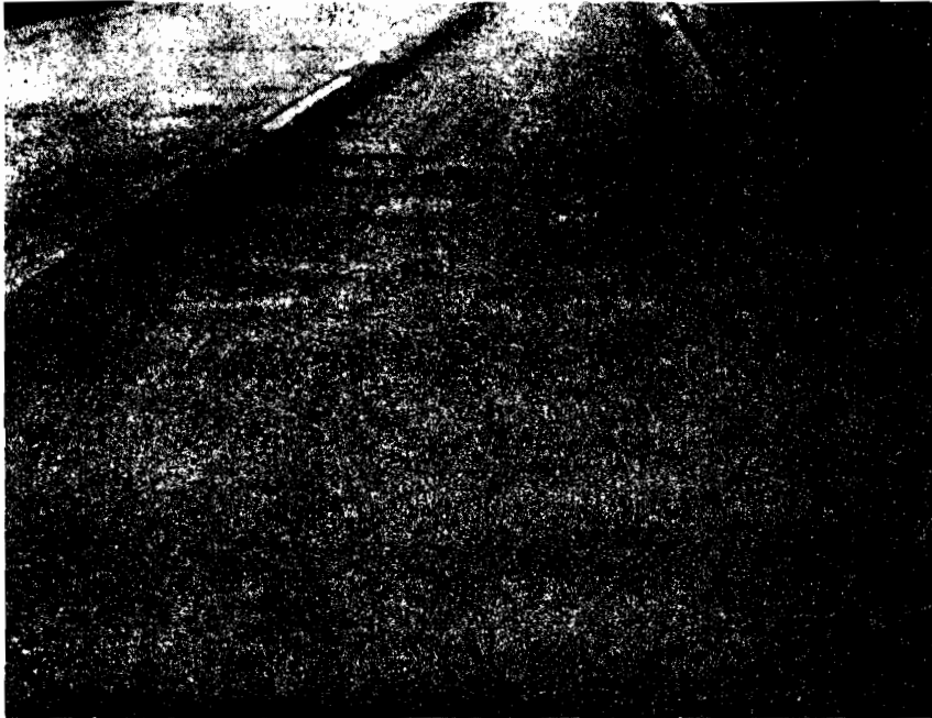
Figure 11 Salt or Sand Spreader Swirled Distribution & Wheel Tracks
