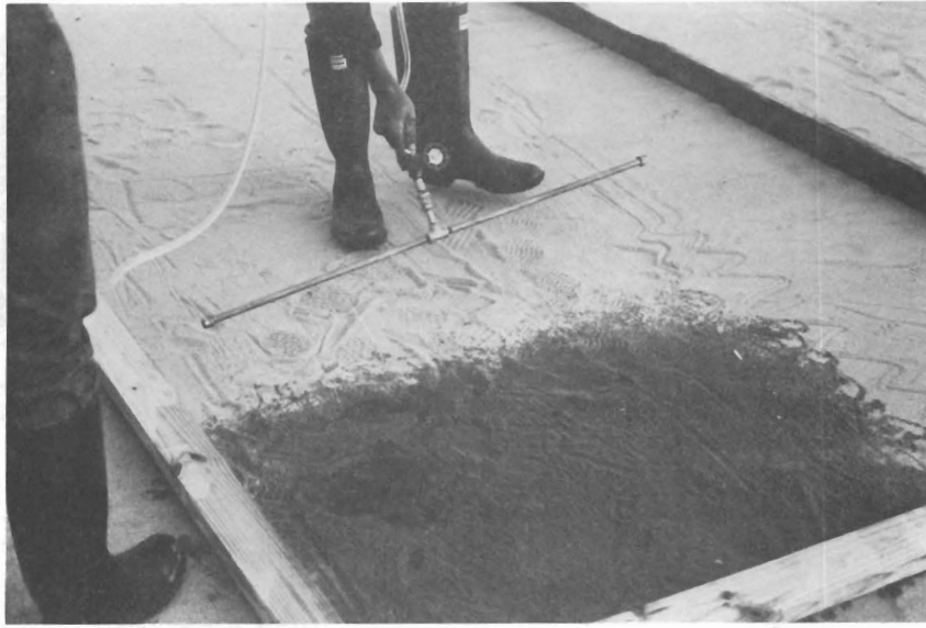
Figure 16 - Application of Monomer to Test Area
