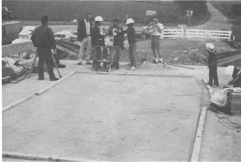
Figure 14 - Screeding the Sand
