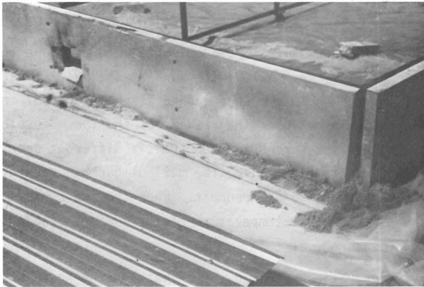
Figure 9 - Sealing Lower Edge of Enclosure with Sand
