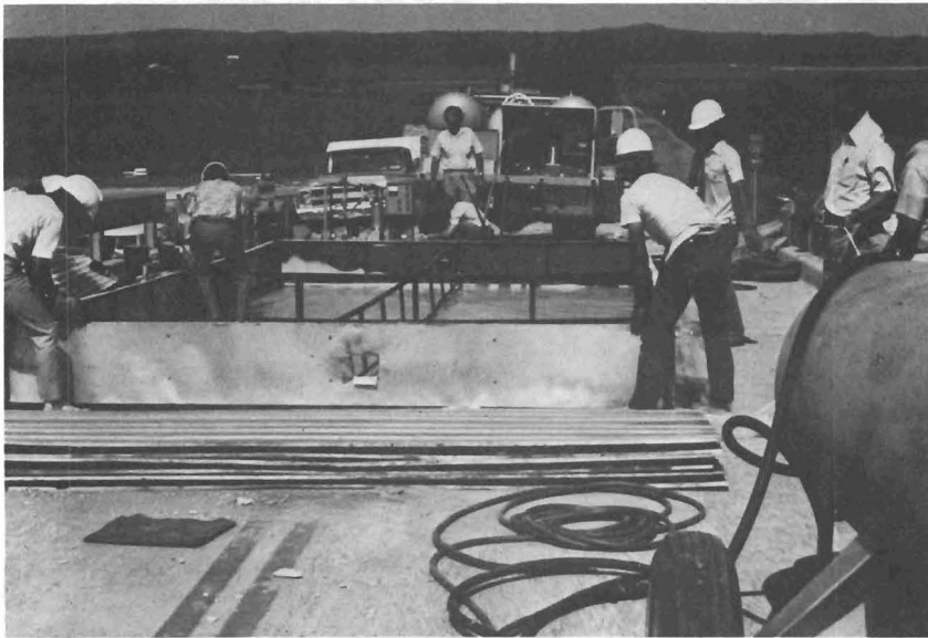
Figure 5 - Installation of Drying Enclosure
