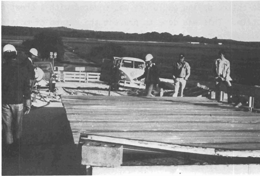
Figure 12 - Cooling the Slab
