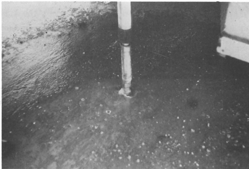
Figure 26 - Coring of Test Area
