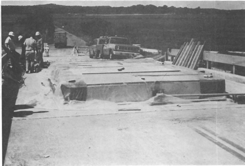
Figure 20 - Enclosure Covered with Polyethylene Sheet
