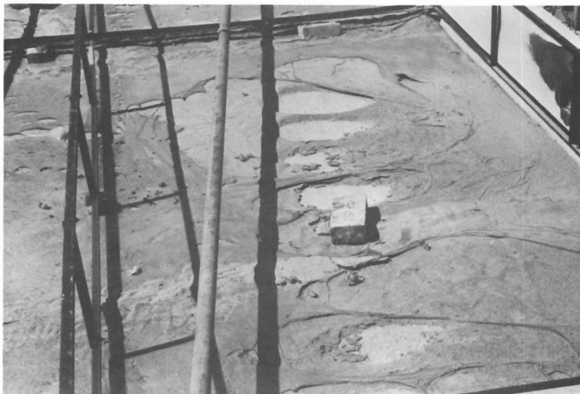
Figure 24 - Exposed Concrete Surface
