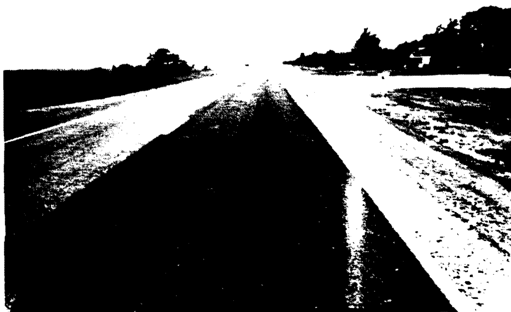
(b) no bleeding distress
