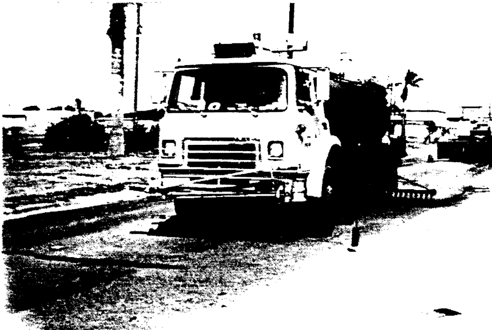
(a) Start of asphalt distribution
