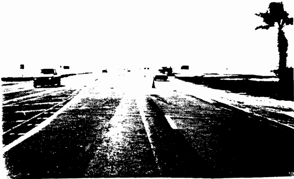
(a) Longitudinal patching in a wheel patch
