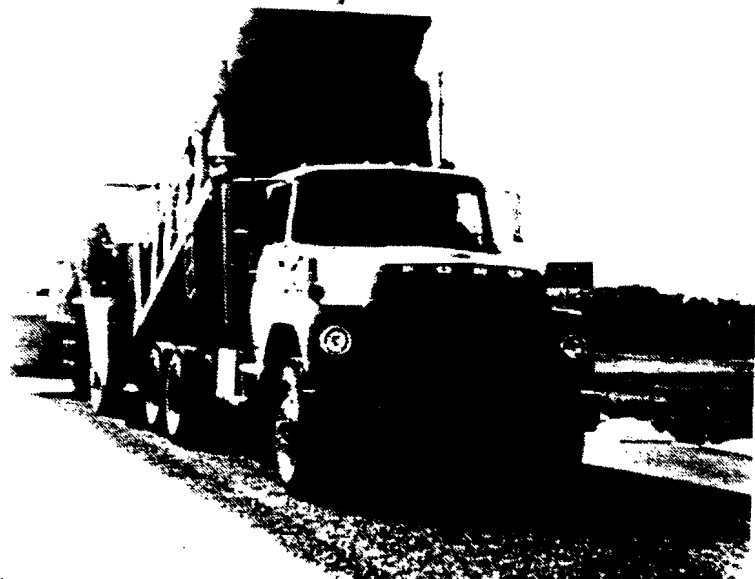
(b) Aggregate spreading in progress
