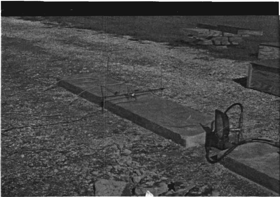
Fig 5.21. Equipment set-up for push-off test No. 1 in Austin, Texas.
