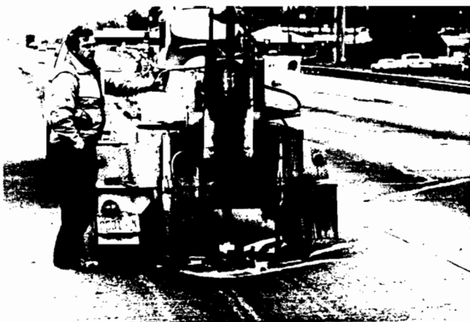
Fig 5.8. Rear view of the coring rig used to retrieve 4-inch-diameter concrete cores for laboratory testing of bond strength.
