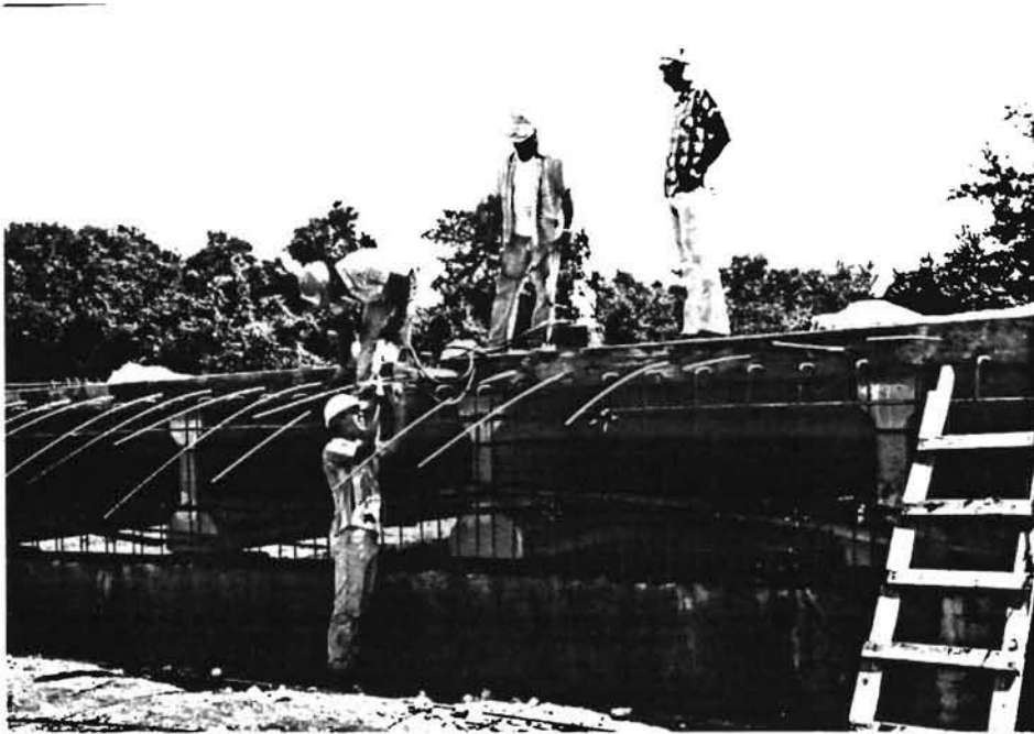
Fig. 2.7 Access to the bottom of the slab at the west end of bridge was possible without the use of platform
