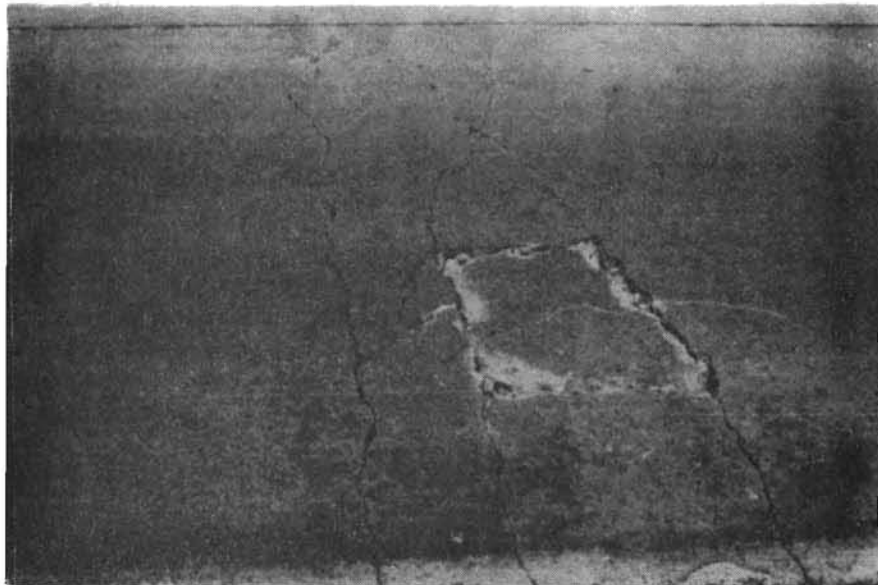
Fig 3. Severe punchouts.
