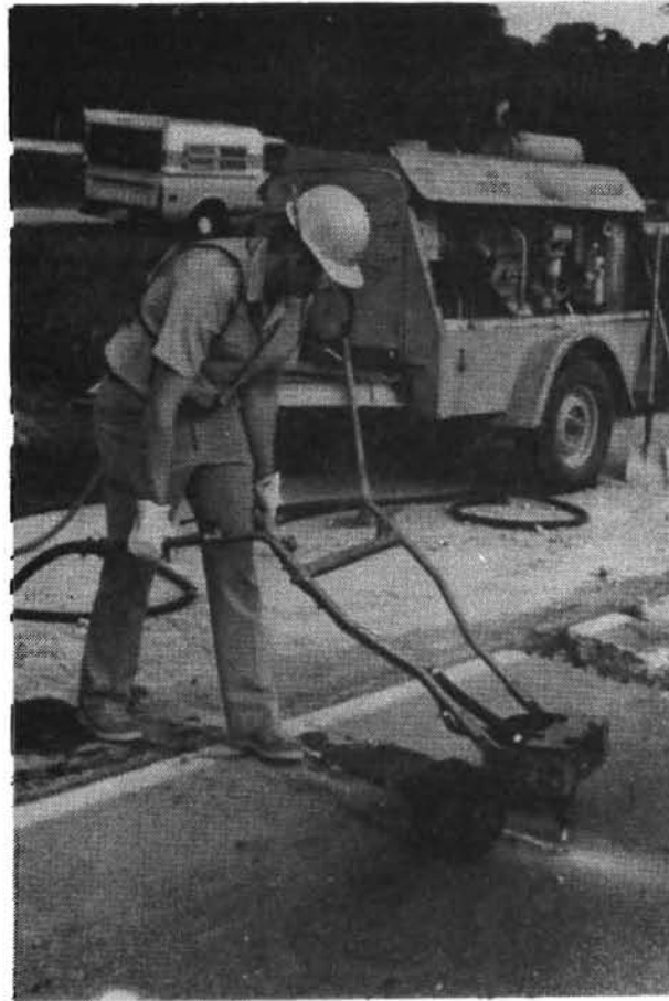
Fig. 2.1 Crack router in operation
