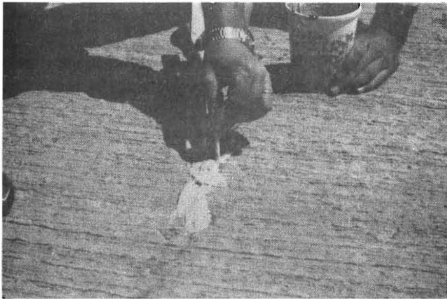
Fig. 5.7 Applying Putty to the Port and Cracks's Surface
