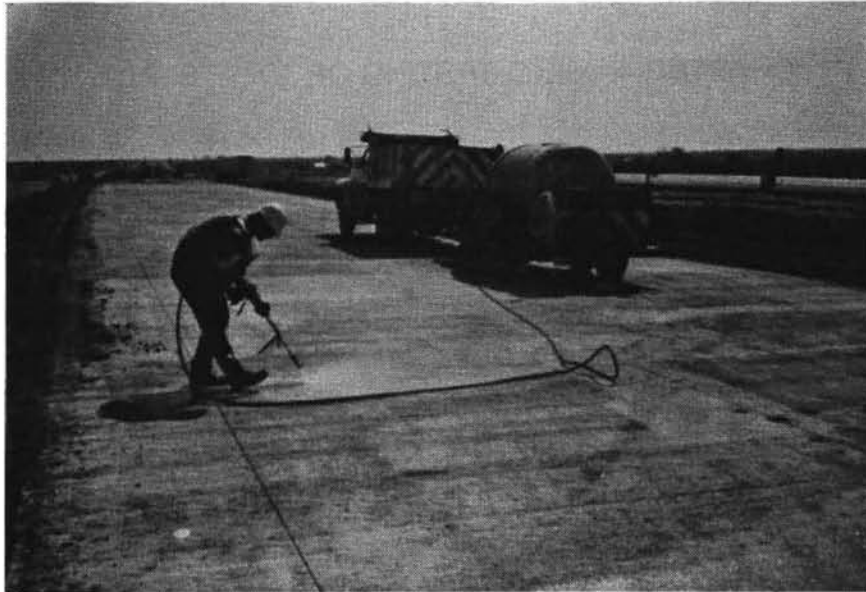
Fig. 4.1 Water Blasting Joints
