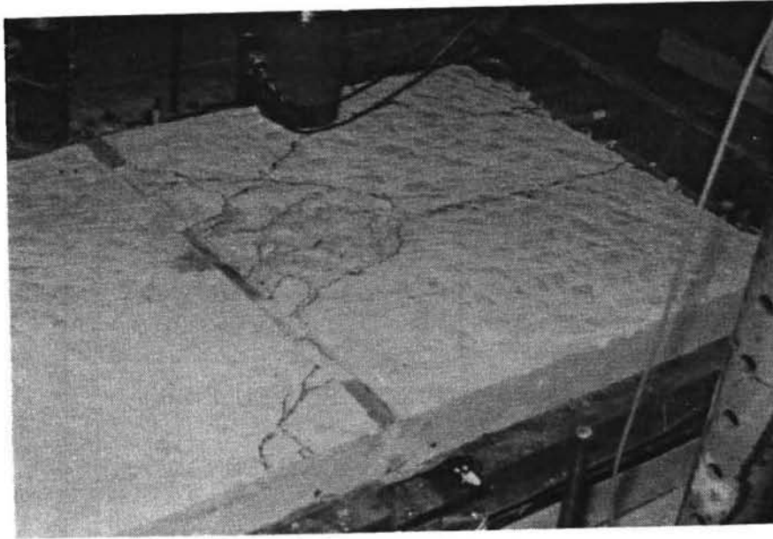
Fig. 3.7 Base Slab with Sealants in Place
