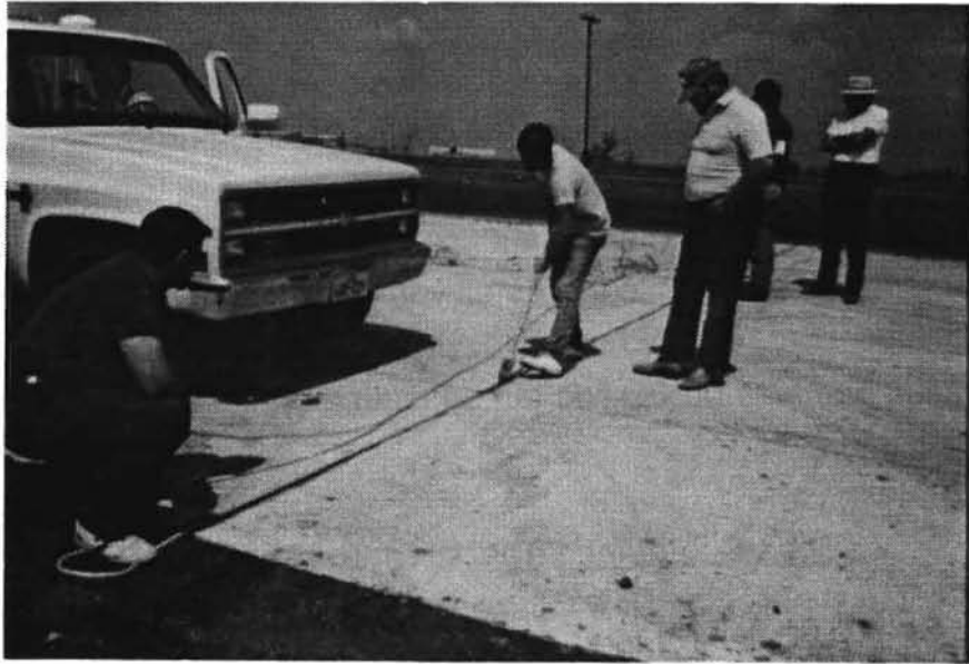
Fig. 4.3 Rolling Backer Rod into Place
