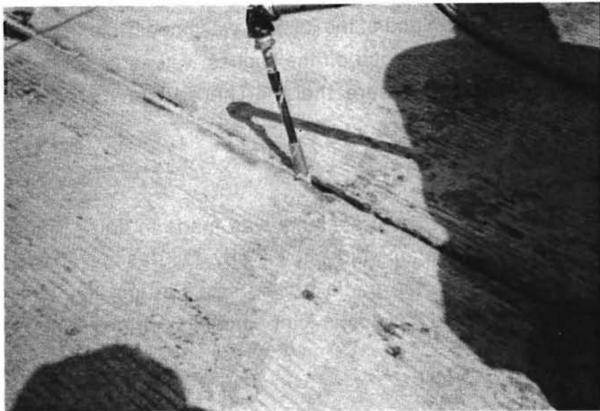
Fig. 4.4 Placing Silicone Sealant
