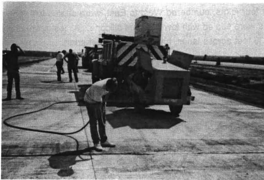
Fig. 4.2 Drying Joints with Compressed Air
