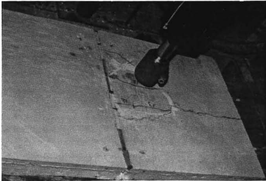
Fig. 3.8 Overlay with Sealants in Place
