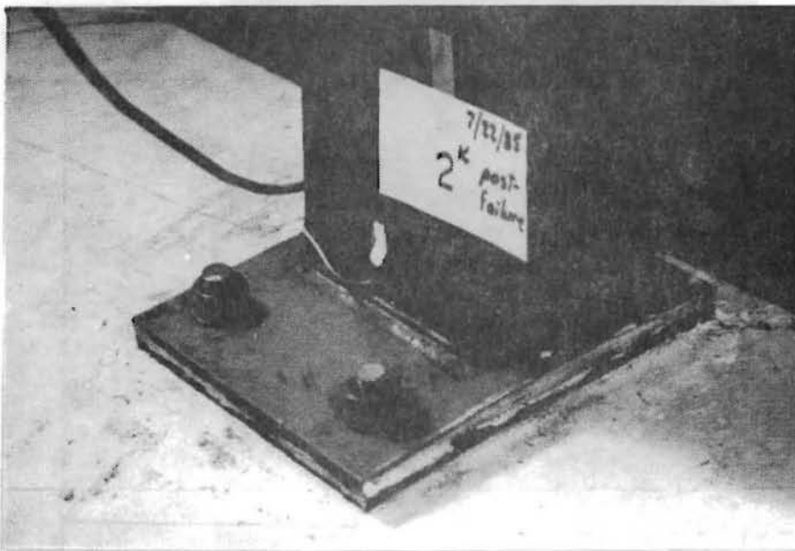
Fig. 5.12 Center post after weld failure
