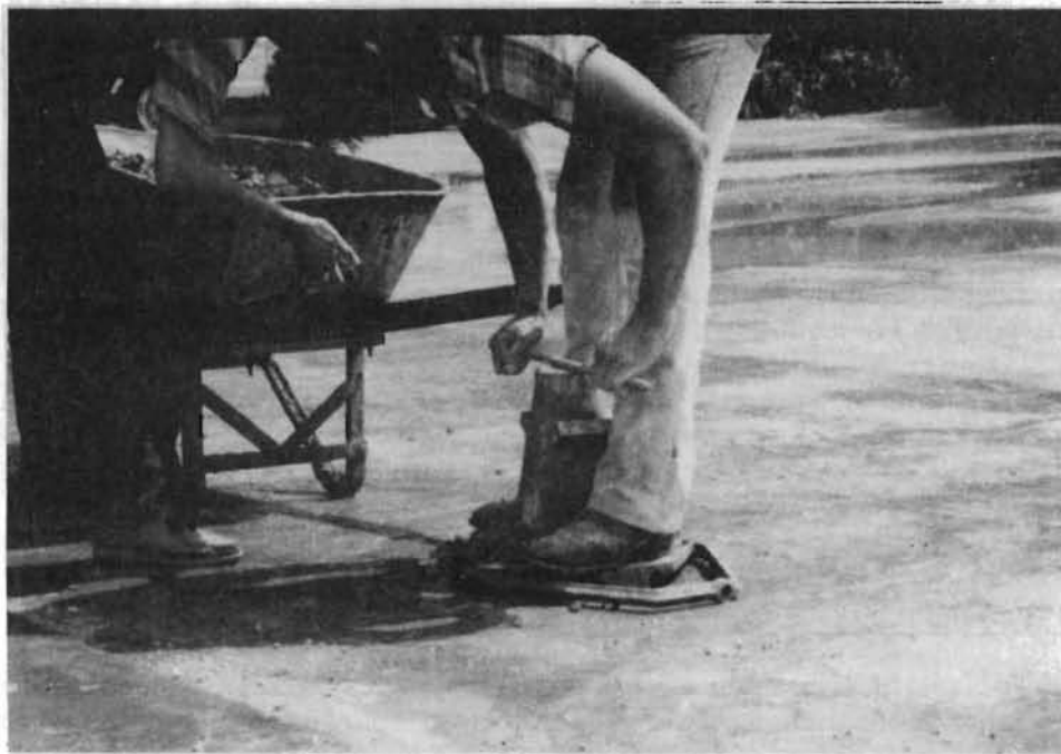
Fig. 3.3 Examination of concrete at ready-mix plant for proper consistency.
