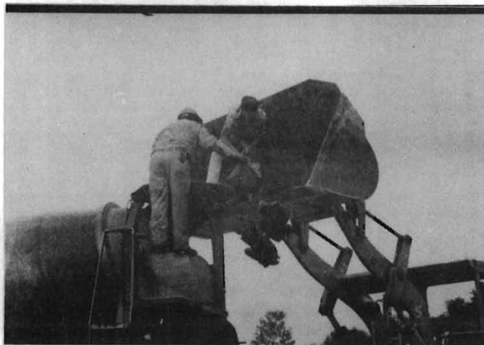
Fig. 3.2 Addition of fly ash to ready-mix truck.
