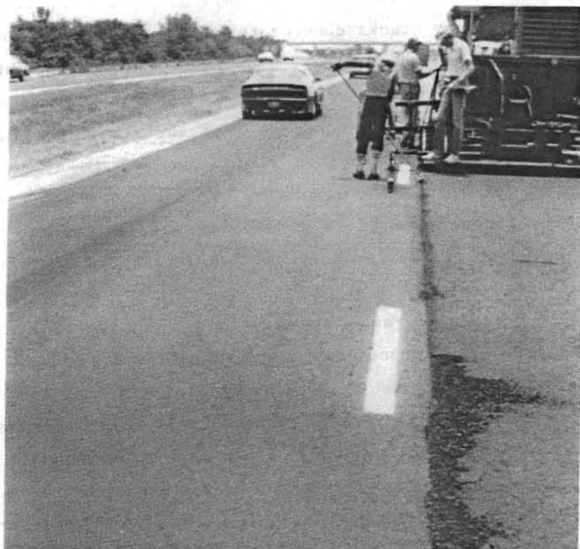
Figure 5.7. Examples of racking the joints
