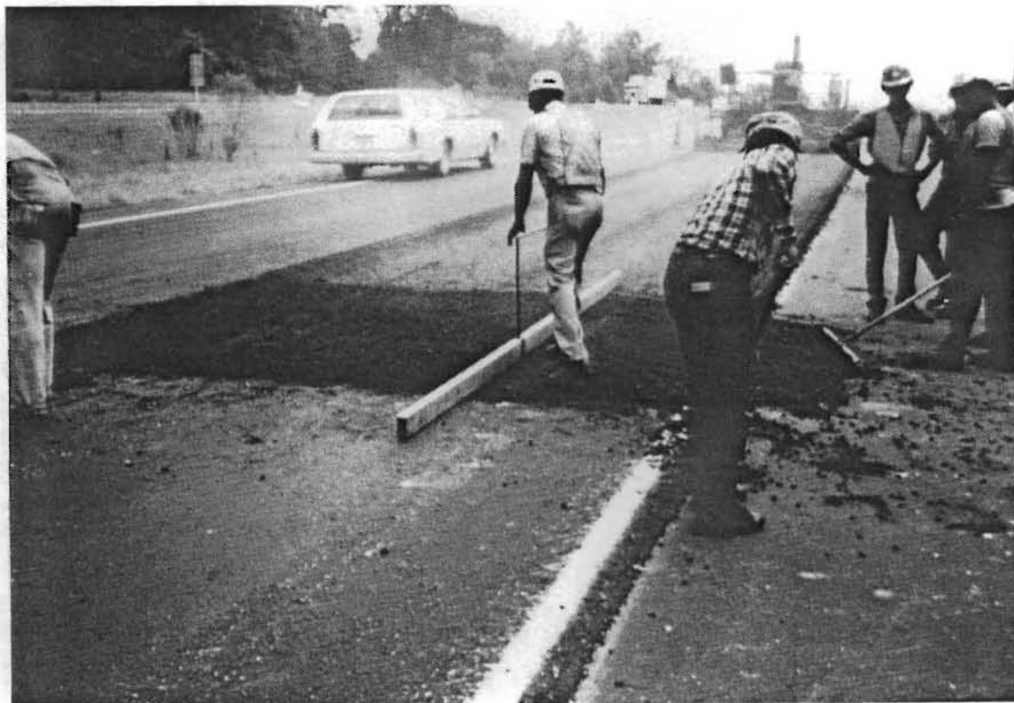
Figure 5.8. Manual placement of hot mix
