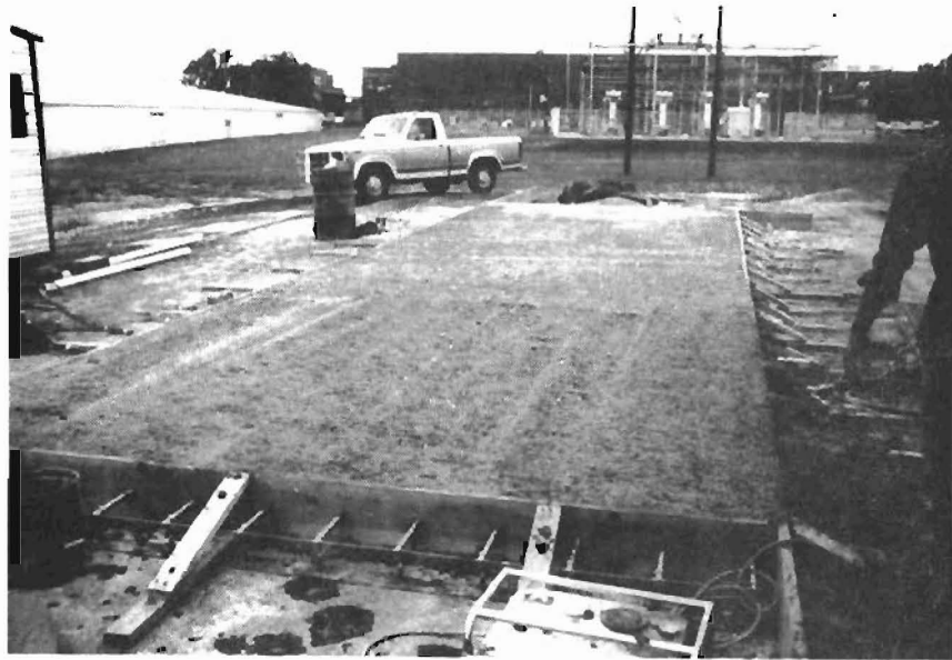
Fig 2.15. Large slab during curing.
