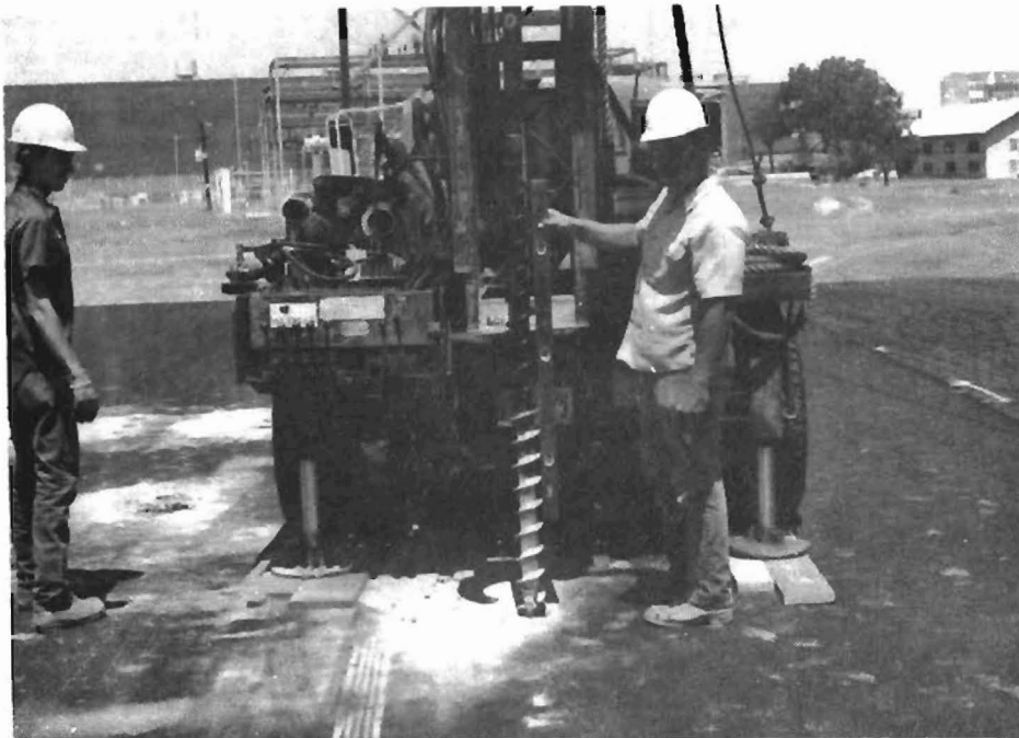
Fig 2.7. Close view of the drilling equipment.
