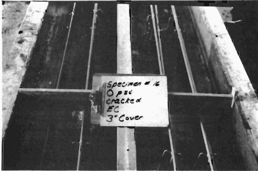
Fig. 3.10 Reinforcement tied to chairs in grouted specimen; wood positioning template in place
