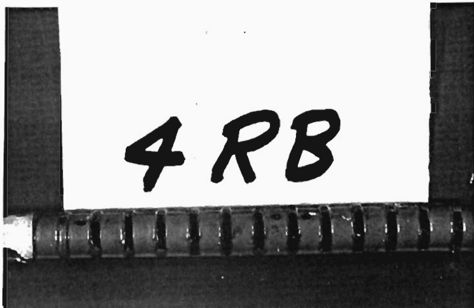
Fig. 4.10 Very light surface corrosion on epoxy-coated reinforcing bar
