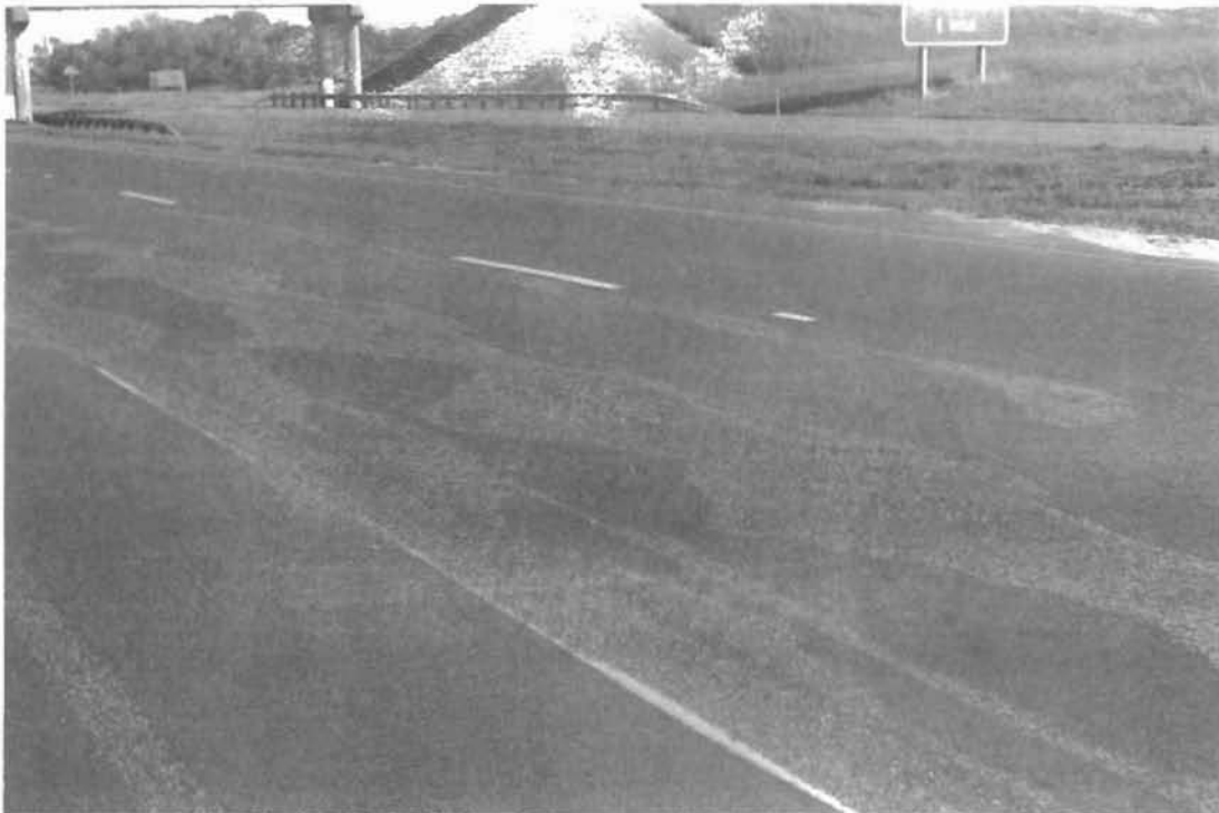
Fig 4. Planing that outlines the longitudinal variation in rutting and shoving distress on IH-10, Columbus.
