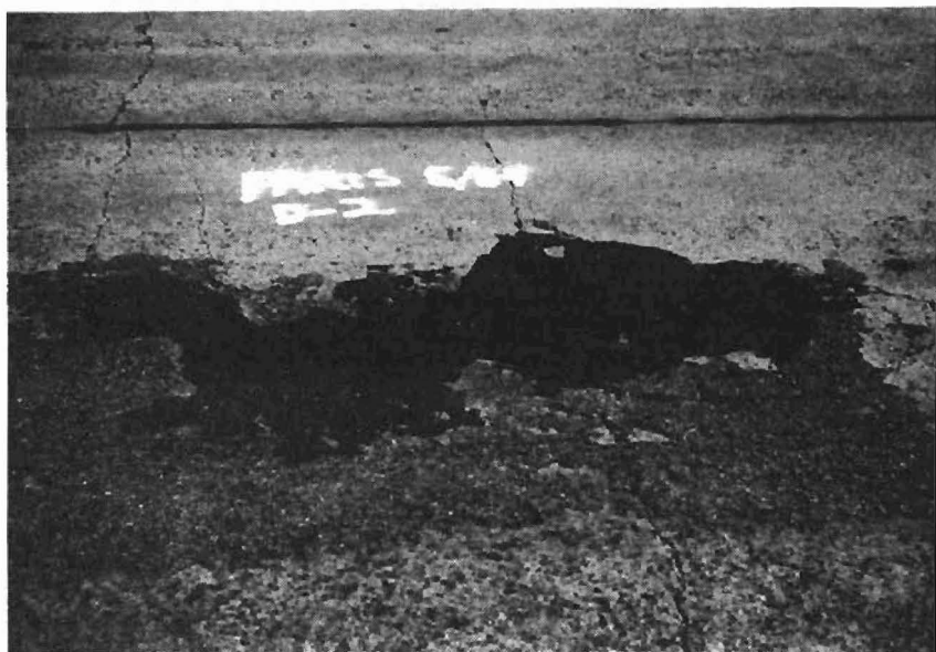
Fig. 7.10. Duracal Repair Area Before Repair
