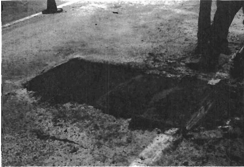
Fig. 7.8. Completed Set-45 Full Depth Repair
