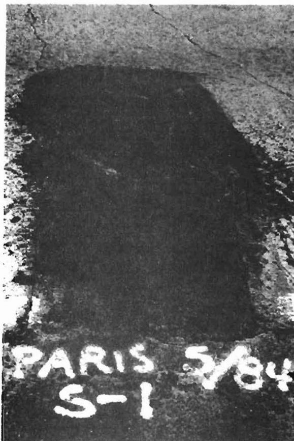
Fig. 7.7. Set-45 Repair Area Before Repair
