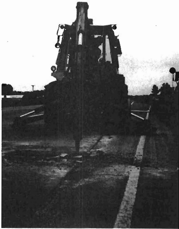
Fig. 7.4. Jackhammering Full Depth Repair
