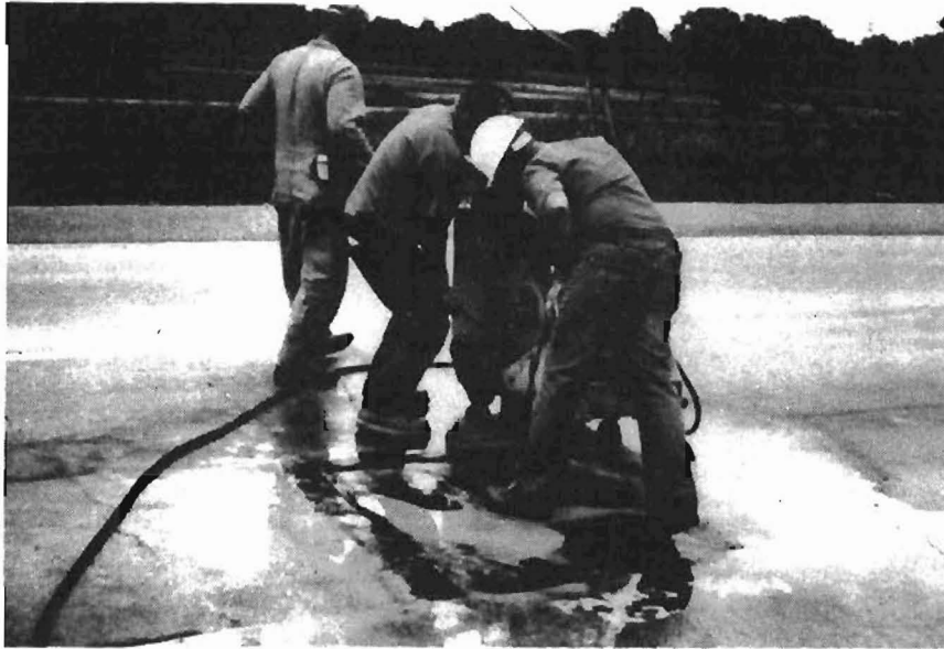
Fig. 7.3. Sawing of Full Depth Repair
