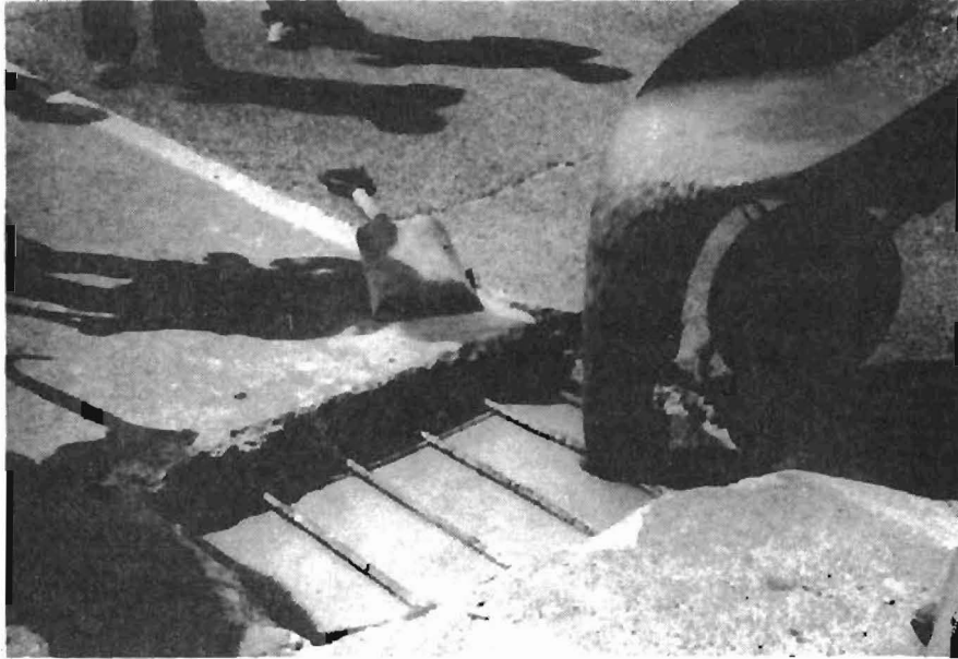
Fig. 7.5. Placing Duracal Repair Mix, Waco.
