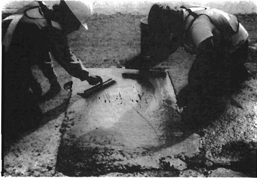
Fig. 7.14. Finishing Duracal Repair, Amarillo.
