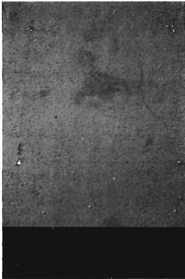
Fig. 7.8. Finished GHP Repair, Waco.
