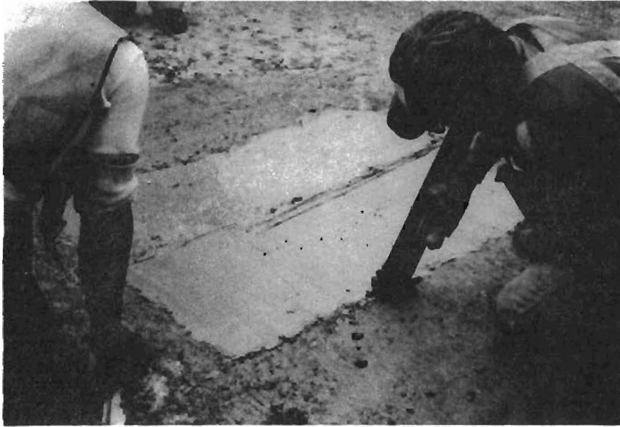
Fig. 7.19. Finishing Duracal Repairs (with and without fibers), Dallas.
