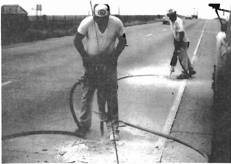
Fig. 7.2. Jack hammering Duracal and GHP Repairs, Waco.
