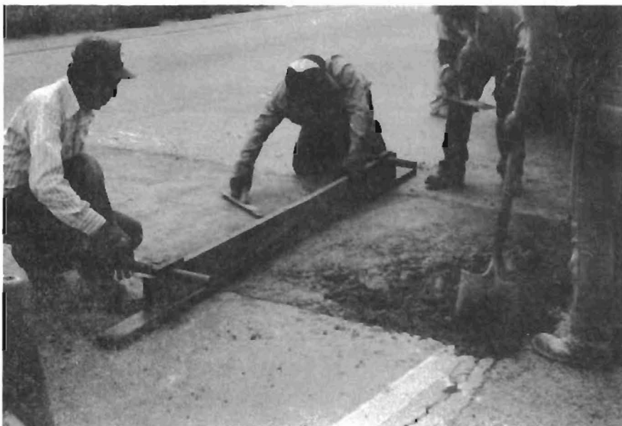
Fig. 6.3. Finishing Class "K" Concrete at Waco.
