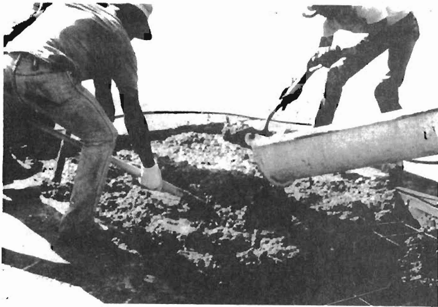
Fig. 6.17. Placing Class "k" Concrete at Houston.
