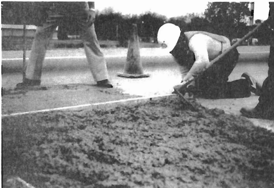
Fig. 6.14. Finishing Class "k" Concrete at Dallas.
