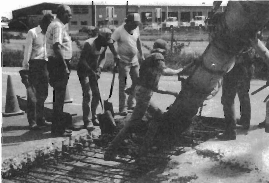
Fig. 6.2. Placing Class "K" Concrete at Waco.
