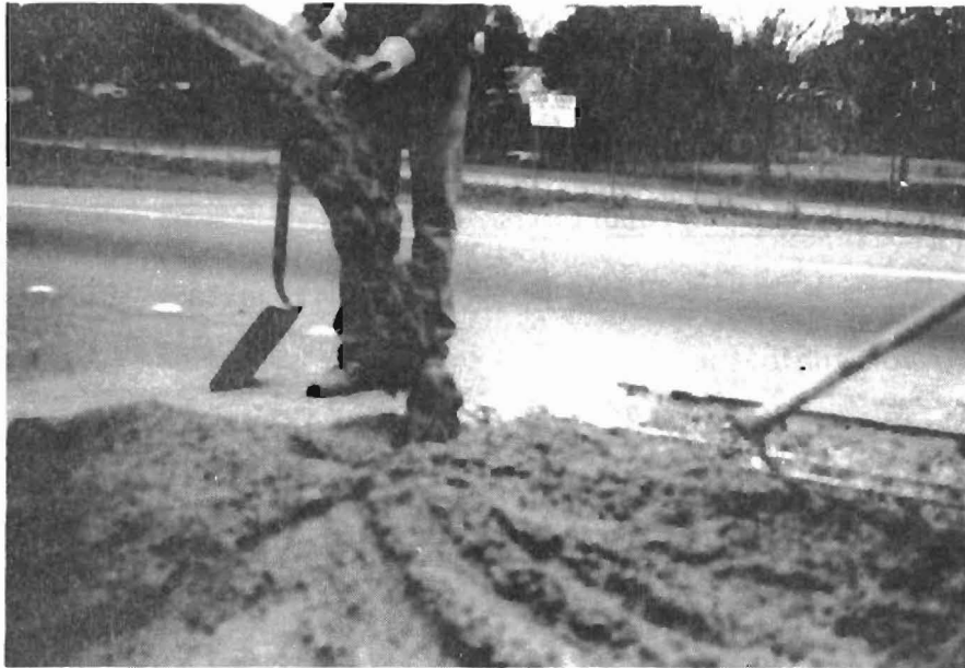
Fig. 6.13. Placing Class "k" Concrete at Dallas.
