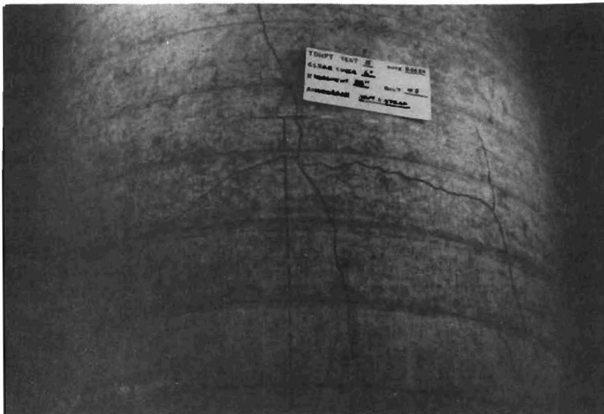
Fig. 7.11 Crack pattern of test SB5
