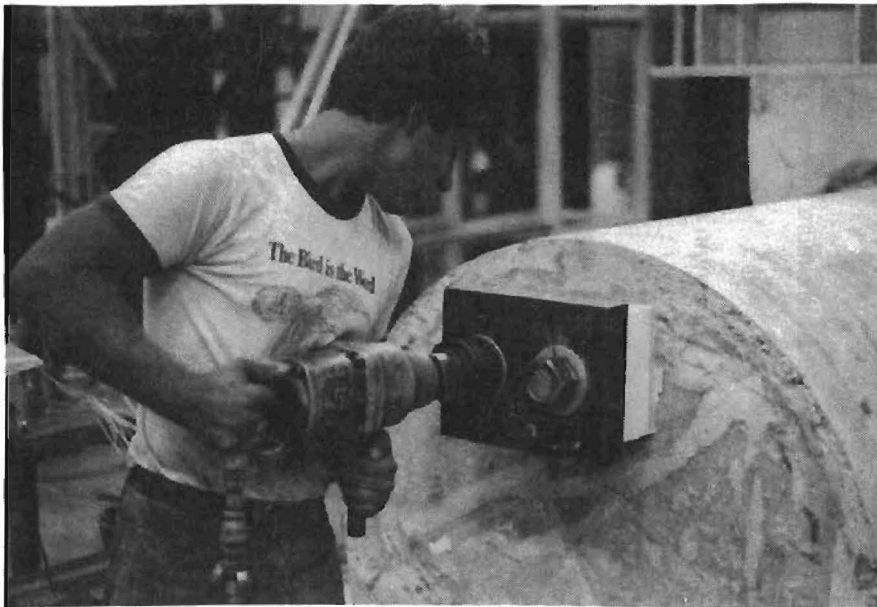
(c) Tightening with pneumatic wrench
