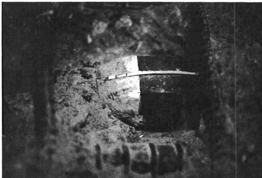
Fig. 4.16 Cone of crushed and compacted concrete in front of anchorage device
