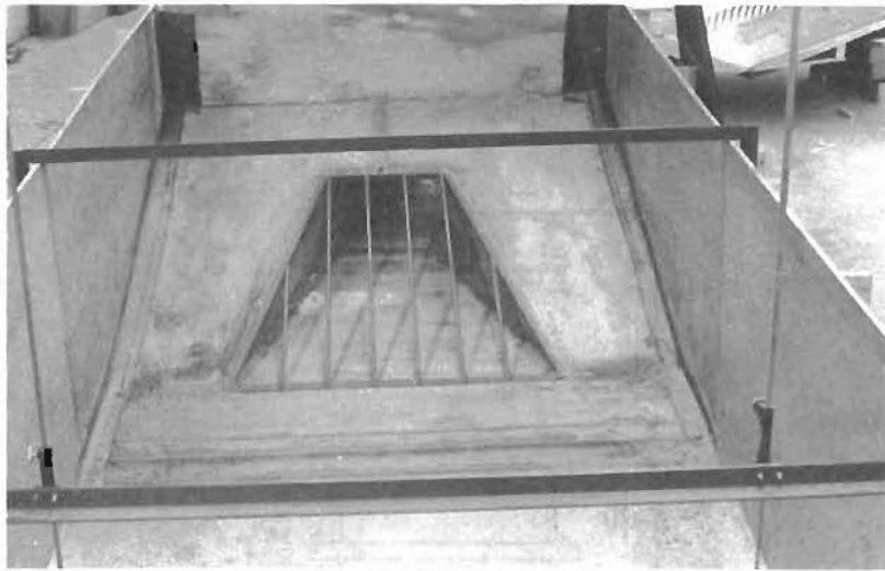
(a) Pipe Safety Grates Installed
