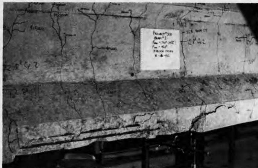
Fig. 4.7 Concrete spalling prior to static ultimate test
