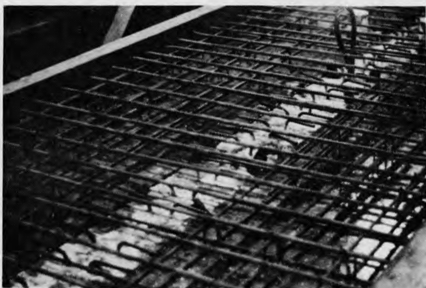
Fig. 3.25 Slab reinforcement
