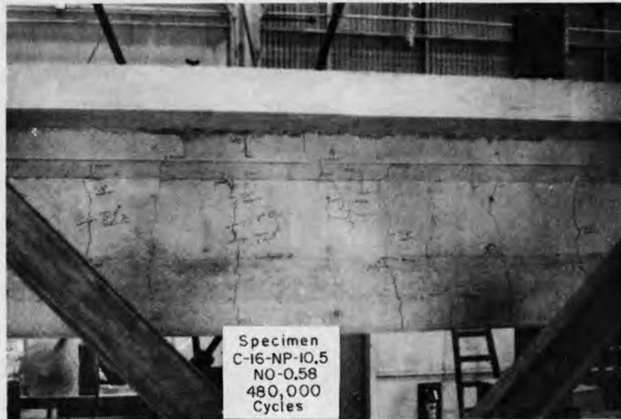
Fig. 4.6 Cracking pattern for Specimen C-16-NP-10.5-NO-0.58 after 480,000 cycles
