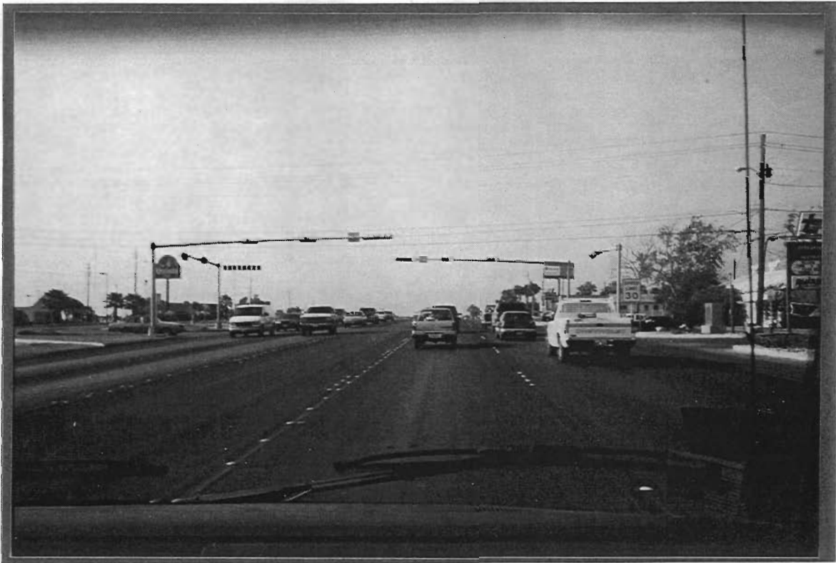
Photo 1. Intersection of US 90 and Cantu
