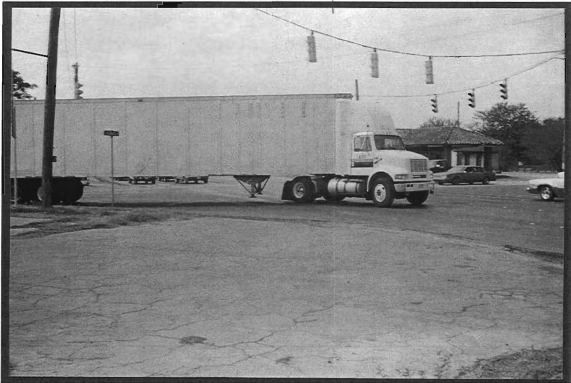
Photo 11. Turning problem at US 90 and Avenue F
