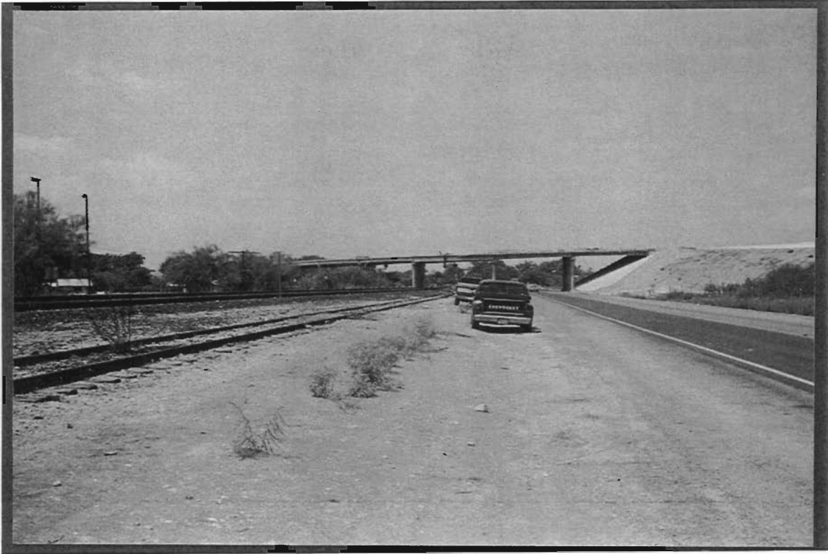
Photo 25. Overpass (new spur)
