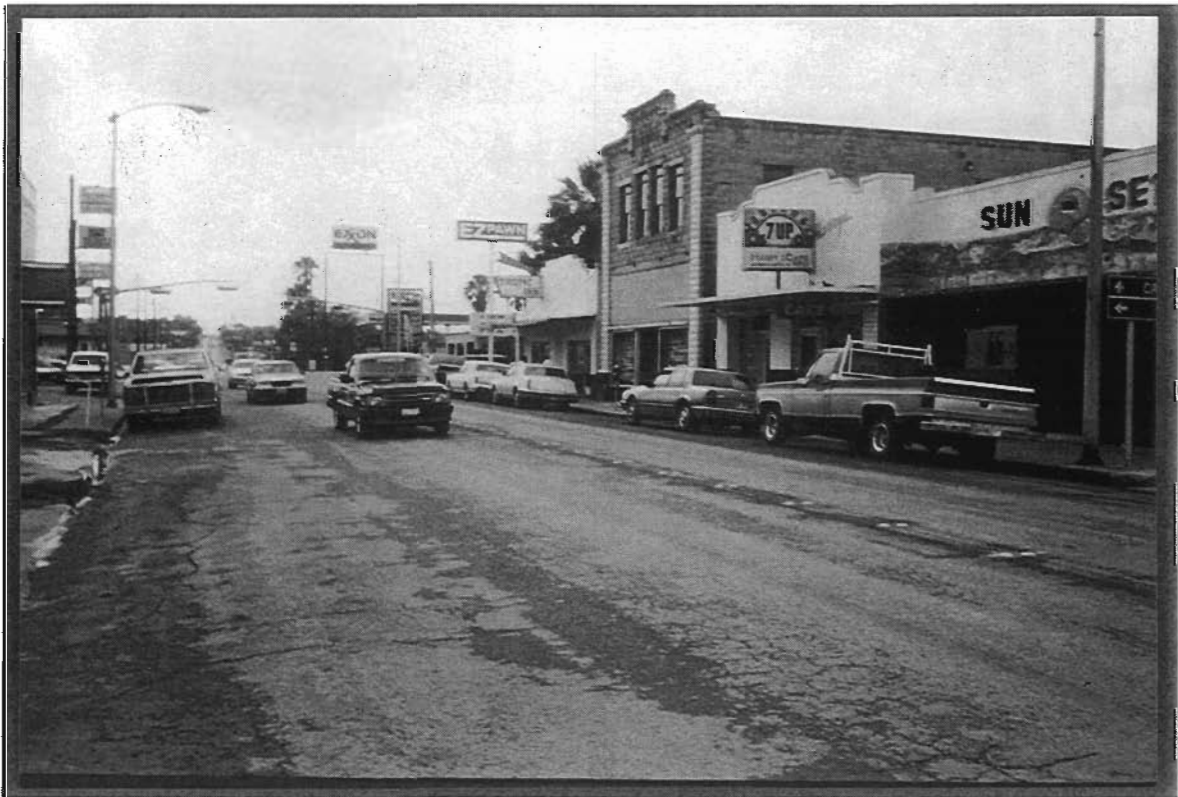
Photo 35. Parking Lanes on Main Street
