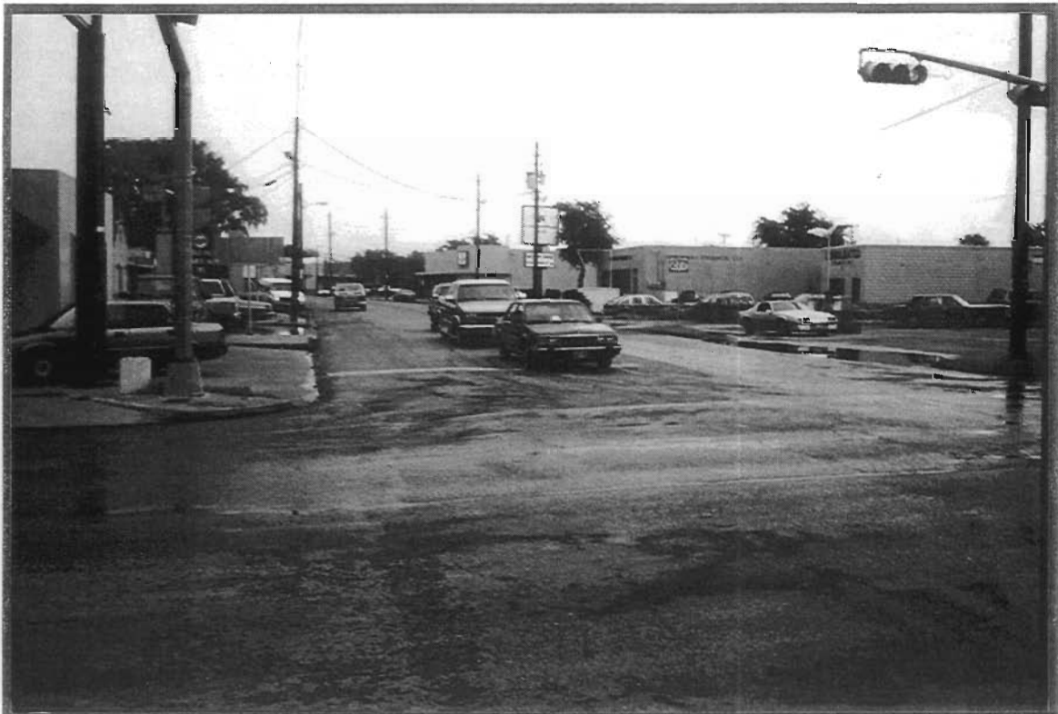
Photo 2. US 277 Business (Ceylon Street) North of Main Street
