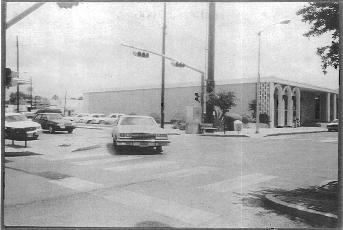
Photo 36. Turning Problem due to Projected Curb along Main Street
