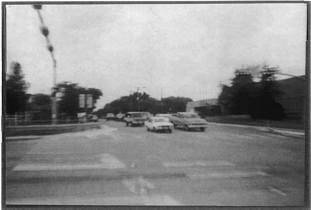
Photo 20. FM 1021 South of US 57 (Near City Hall)
