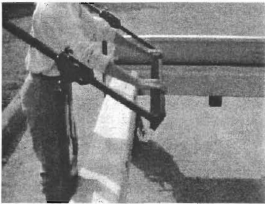
Figure 11.3 Lifting the Canopy
