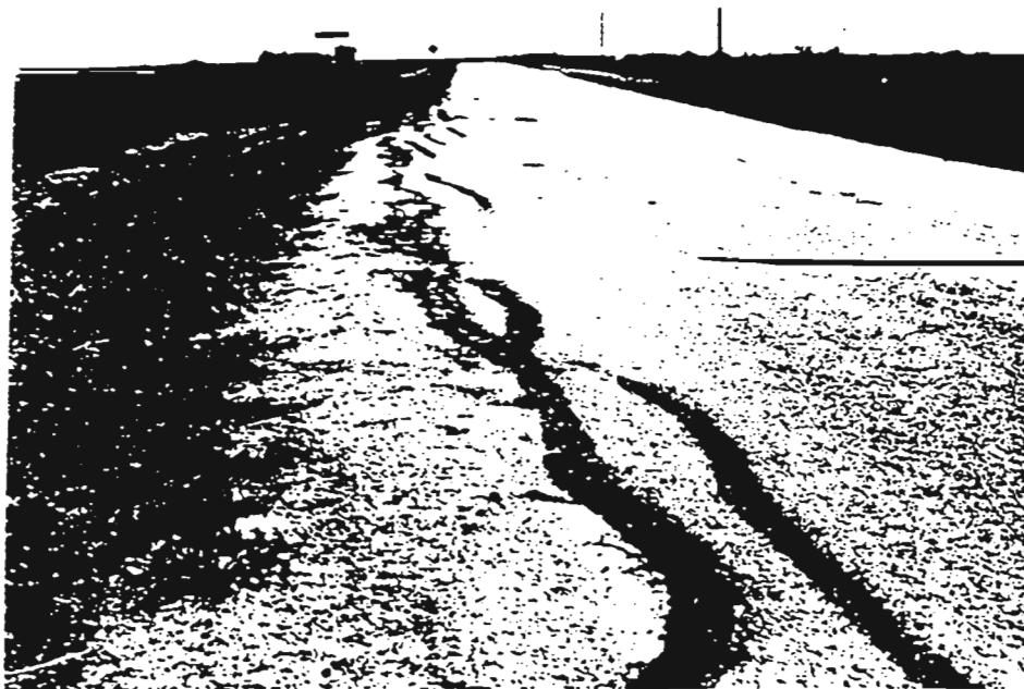
Figure 4.1 Asphalt Concrete Cracks Sealed by Maintenance Crews
