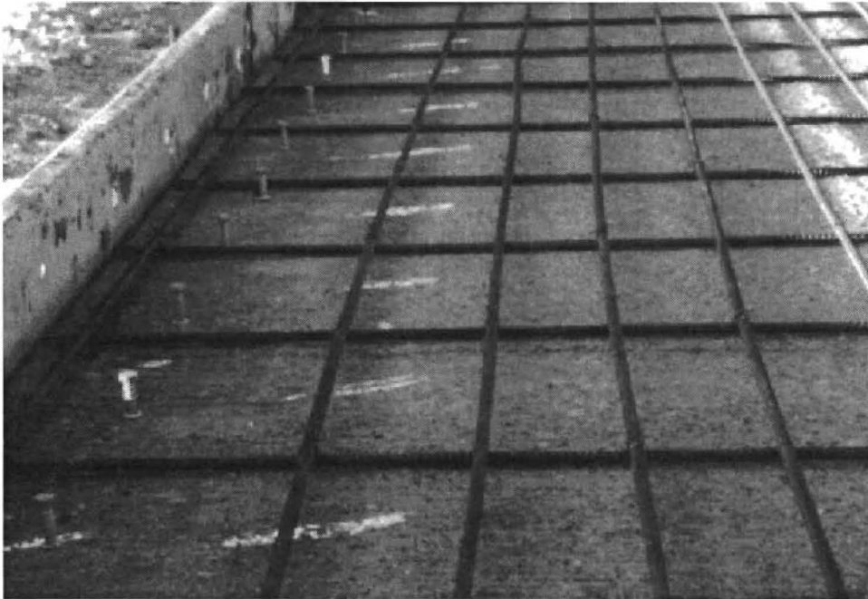
Figure 4.3 Installed nails and reinforcement with formwork
