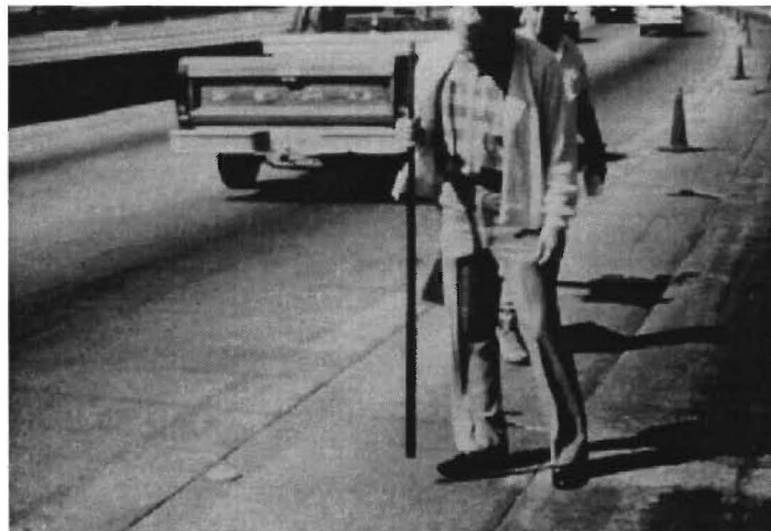
Figure 4.17 Rebar sounding
