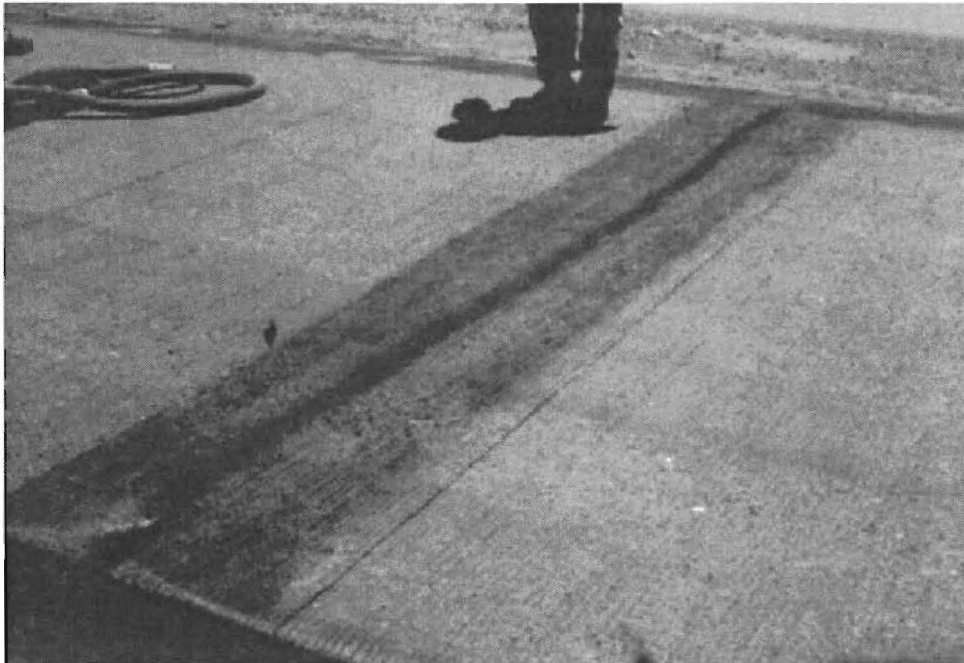
Figure 4.6 Debonding agent between sections
