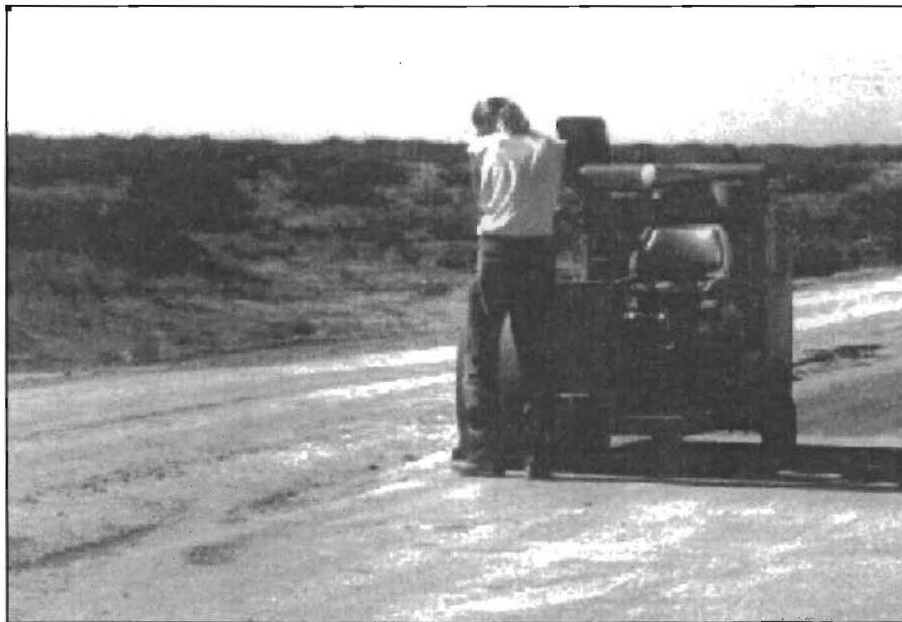
Figure 4.5 Shotblasting equipment used
